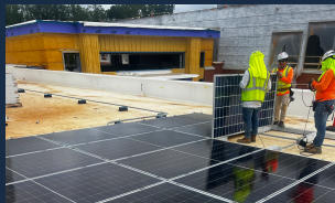
Solar panel delivery & install
