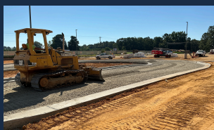
ABC stone placement and grading
