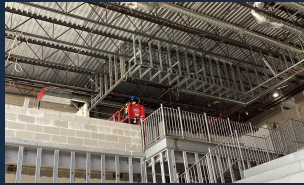
2nd floor soffit framing (Area A)
