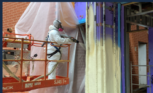
Entry spray foam (Area A)
