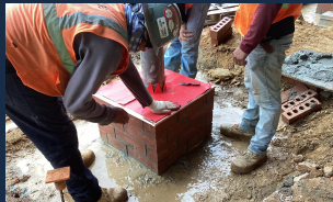
Brick veneer column wrap & flashing
