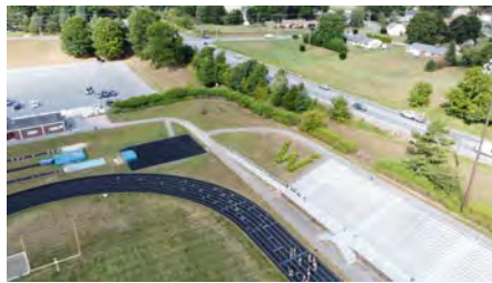
Photo #17 (Westminster Aerial Overall (17).JPG)
