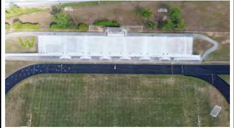
Photo #3 (Westminster Aerial Overall (3).JPG)
