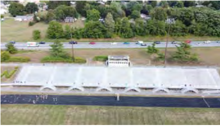
Photo #1 (Westminster Aerial Overall (1).JPG)
