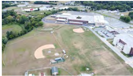
Photo #8 (Westminster Aerial Overall (8).JPG)
