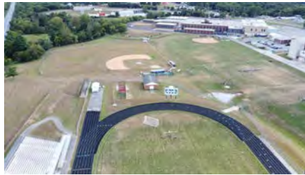
Photo #14 (Westminster Aerial Overall (14).JPG)
