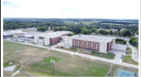
Photo #15 (Westminster Aerial Overall (15).JPG)
