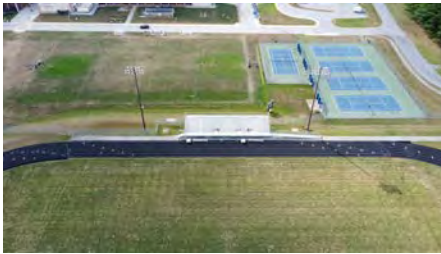
Photo #13 (Westminster Aerial Overall (13).JPG)
