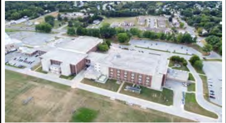
Photo #6 (Westminster Aerial Overall (6).JPG)
