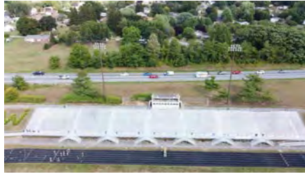
Photo #2 (Westminster Aerial Overall (2).JPG)
