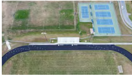
Photo #5 (Westminster Aerial Overall (5).JPG)
