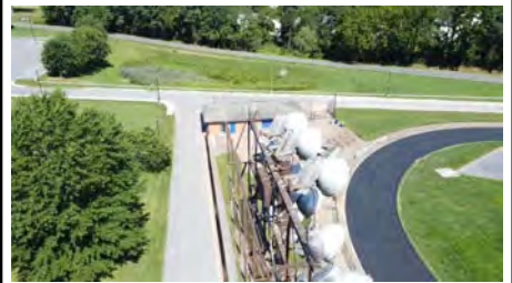
Photo #81 (Liberty Aerial W4 (81).JPG)
