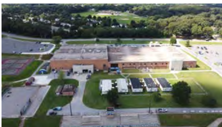
Photo #7 (Liberty Aerial Overall (7).JPG)
