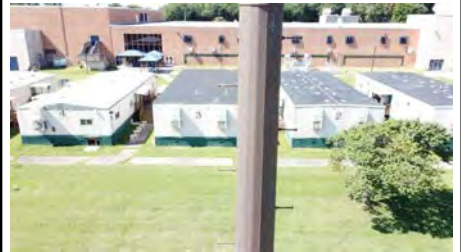
Photo #60 (Liberty Aerial W4 (60).JPG)
