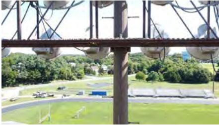
Photo #19 (Liberty Aerial W4 (19).JPG)
