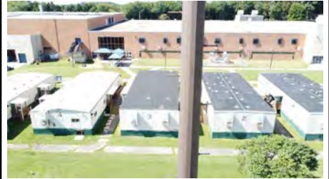
Photo #66 (Liberty Aerial W4 (66).JPG)
