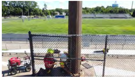
Photo #2 (Liberty Aerial W4 (2).JPG)
