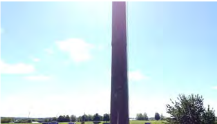
Photo #49 (Liberty Aerial W4 (49).JPG)
