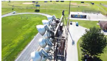
Photo #32 (Liberty Aerial W4 (32).JPG)
