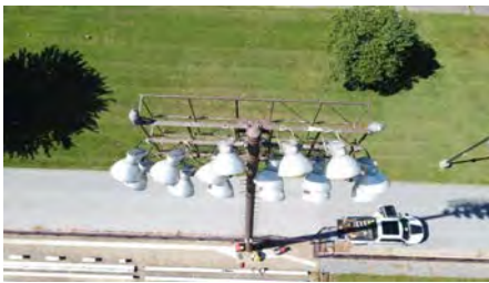
Photo #79 (Liberty Aerial W4 (79).JPG)
