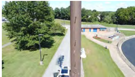
Photo #95 (Liberty Aerial W4 (95).JPG)
