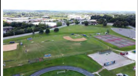
Photo #9 (Liberty Aerial Overall (9).JPG)
