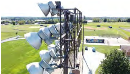
Photo #34 (Liberty Aerial W4 (34).JPG)
