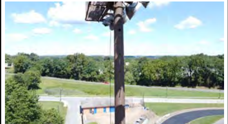
Photo #87 (Liberty Aerial W4 (87).JPG)
