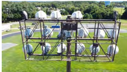
Photo #23 (Liberty Aerial W4 (23).JPG)
