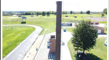
Photo #45 (Liberty Aerial W4 (45).JPG)
