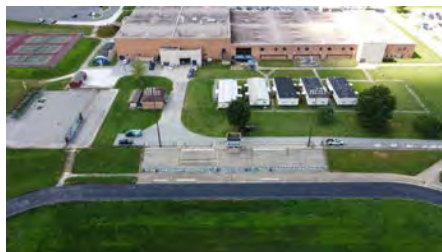
Photo #5 (Liberty Aerial Overall (5).JPG)
