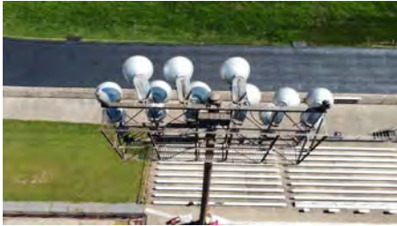
Photo #28 (Liberty Aerial W4 (28).JPG)
