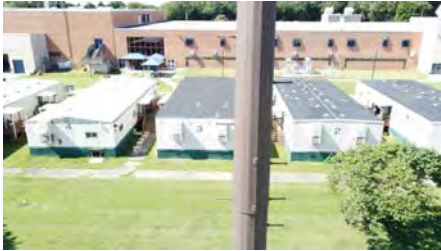
Photo #64 (Liberty Aerial W4 (64).JPG)
