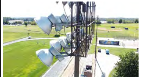
Photo #36 (Liberty Aerial W4 (36).JPG)
