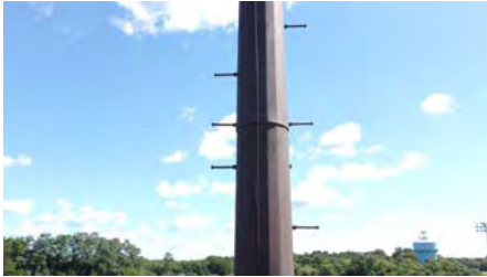
Photo #10 (Liberty Aerial W4 (10).JPG)
