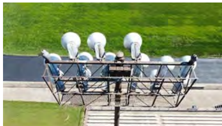
Photo #26 (Liberty Aerial W4 (26).JPG)
