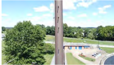
Photo #92 (Liberty Aerial W4 (92).JPG)
