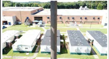
Photo #69 (Liberty Aerial W4 (69).JPG)
