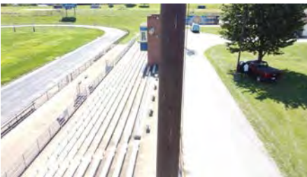
Photo #52 (Liberty Aerial W4 (52).JPG)
