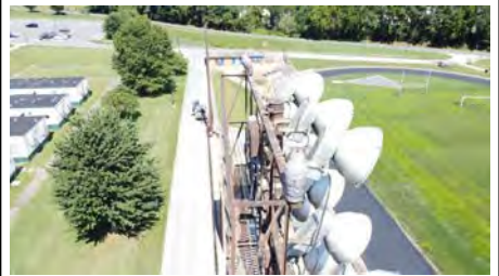
Photo #36 (Liberty Aerial S3 (36).JPG)
