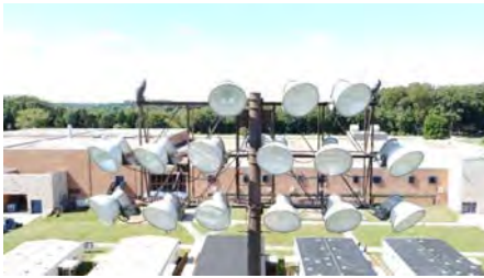
Photo #76 (Liberty Aerial W4 (76).JPG)
