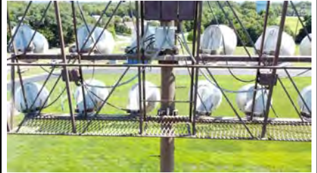
Photo #21 (Liberty Aerial W4 (21).JPG)
