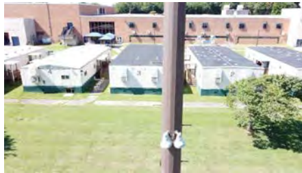
Photo #59 (Liberty Aerial W4 (59).JPG)
