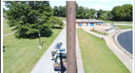
Photo #96 (Liberty Aerial W4 (96).JPG)
