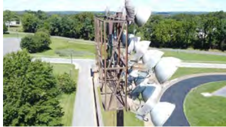
Photo #83 (Liberty Aerial W4 (83).JPG)
