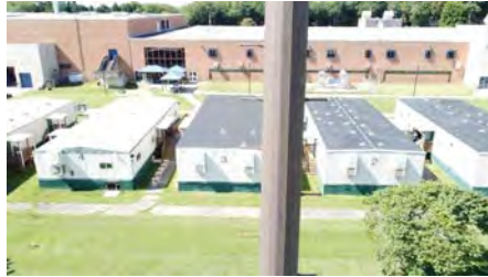
Photo #65 (Liberty Aerial W4 (65).JPG)
