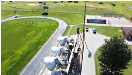
Photo #31 (Liberty Aerial W4 (31).JPG)
