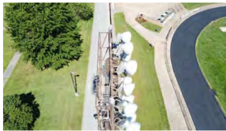
Photo #80 (Liberty Aerial W4 (80).JPG)
