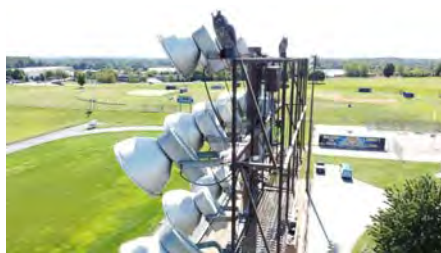
Photo #35 (Liberty Aerial W4 (35).JPG)
