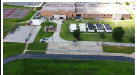
Photo #6 (Liberty Aerial Overall (6).JPG)
