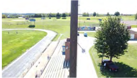
Photo #47 (Liberty Aerial W4 (47).JPG)
