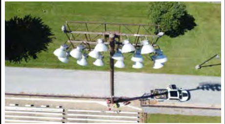
Photo #78 (Liberty Aerial W4 (78).JPG)
