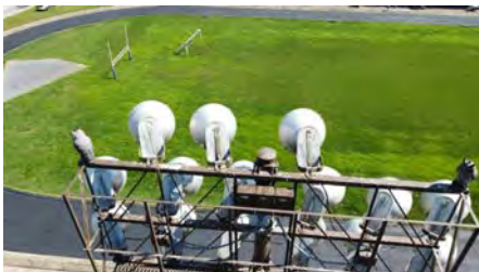
Photo #25 (Liberty Aerial W4 (25).JPG)
