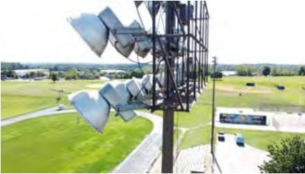
Photo #37 (Liberty Aerial W4 (37).JPG)
