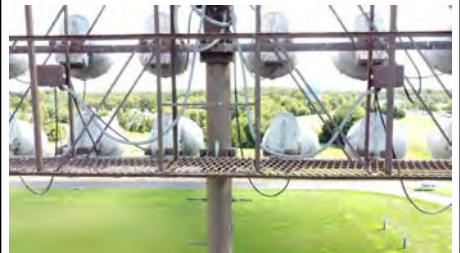
Photo #72 (Liberty Aerial S3 (72).JPG)
