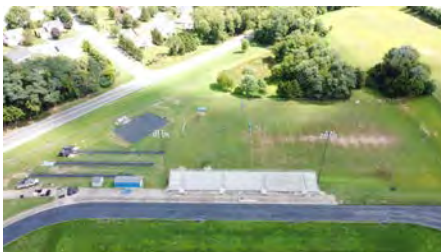
Photo #4 (Liberty Aerial Overall (4).JPG)
