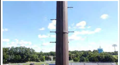
Photo #9 (Liberty Aerial W4 (9).JPG)
