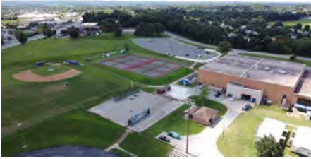
Photo #10 (Liberty Aerial Overall (10).JPG)
