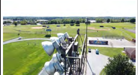
Photo #33 (Liberty Aerial W4 (33).JPG)
