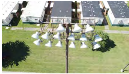
Photo #77 (Liberty Aerial W4 (77).JPG)
