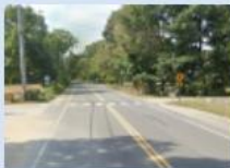
Black Point Road (South)
