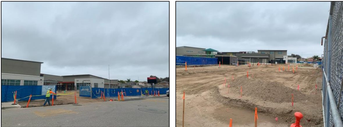
Rose Avenue Elementary School Construction Progress
