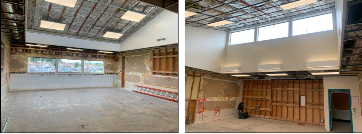
Ritchen Elementary School Construction Progress
