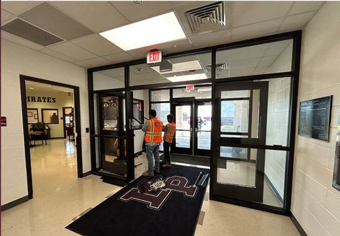
Photo 02 - New storefront installed at middle school
