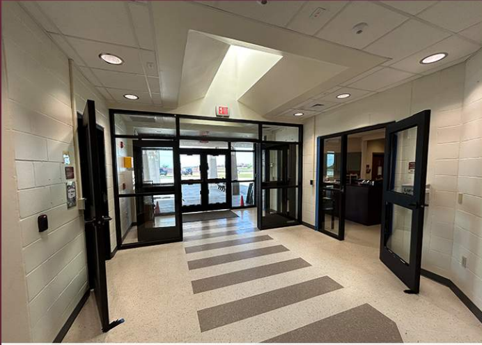
Photo 01 - New storefront installed at high school
