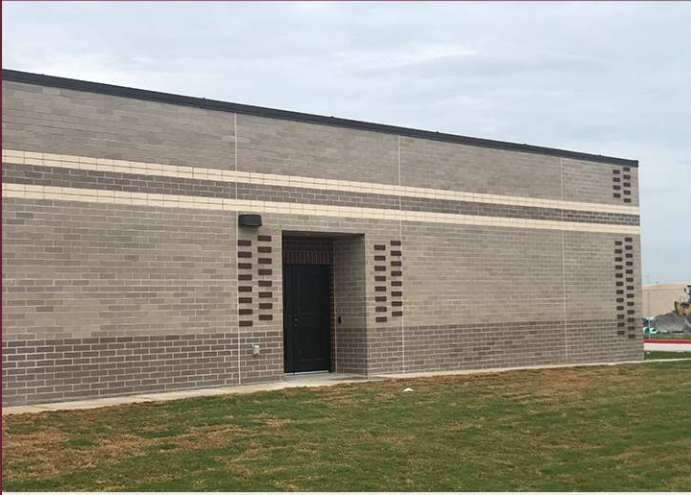
Photo 01 - View south, exterior masonry completed and sod placed
