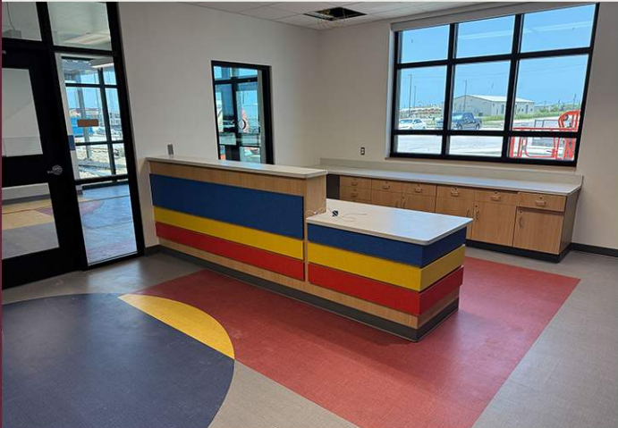
Photo 03 - Interior view at reception, front desk and flooring completed
