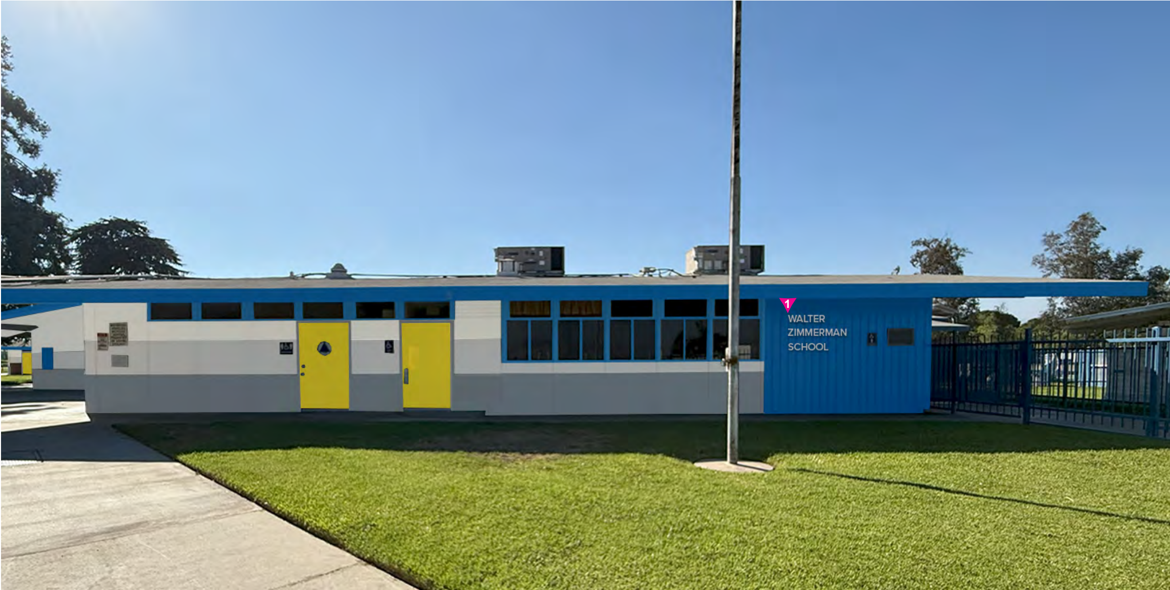
Bldg. 100, Main Office (South Wall / North View)
