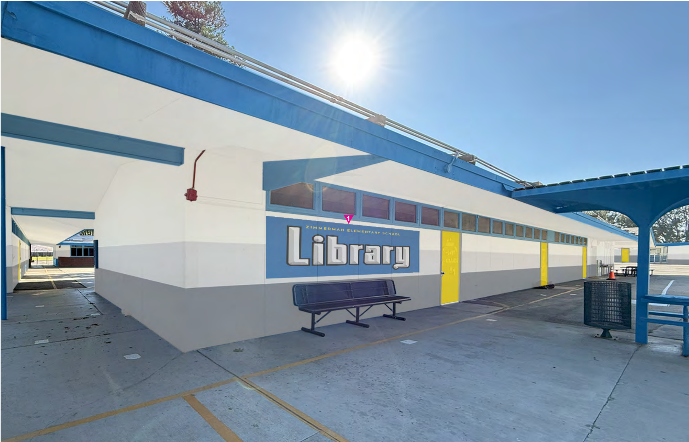
Bldg. 600W - Typical CR (Campus Center)
