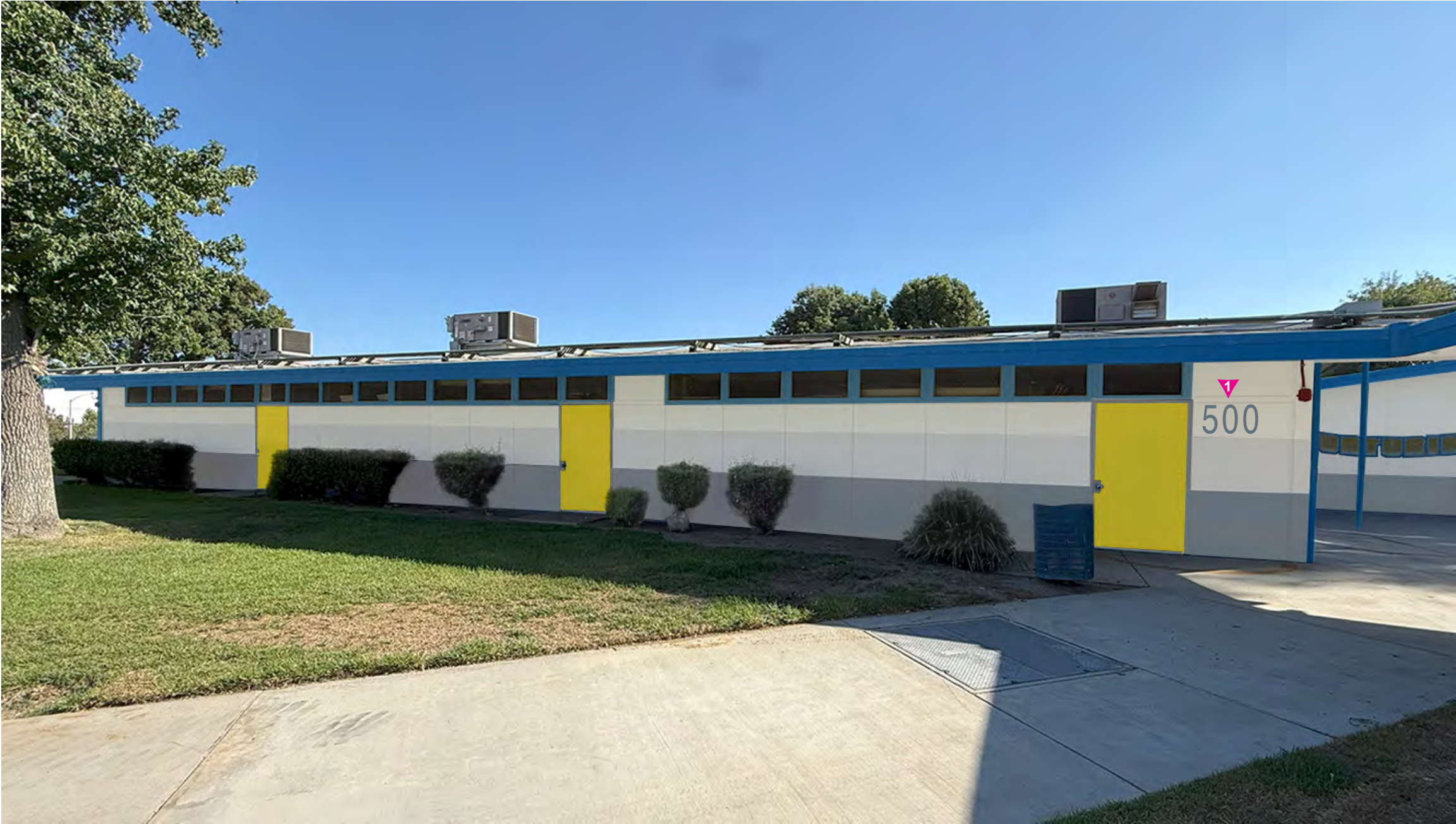
Bldg. 300 - Typical CR (South Wall / West View)
