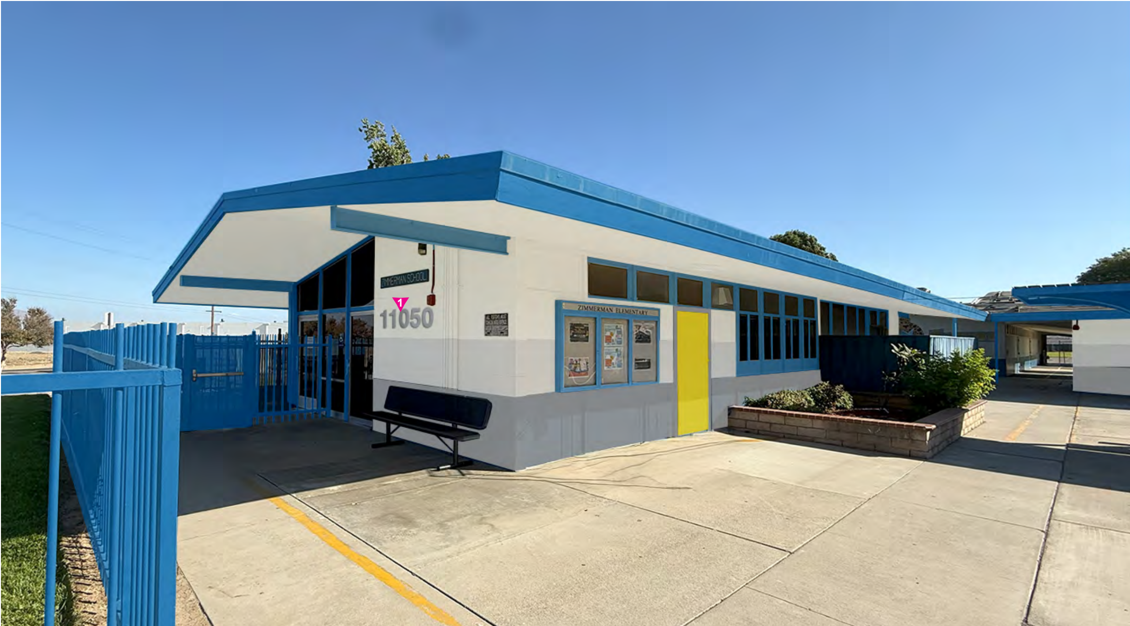
Bldg. 100, Main Office (North Wall / South View)
