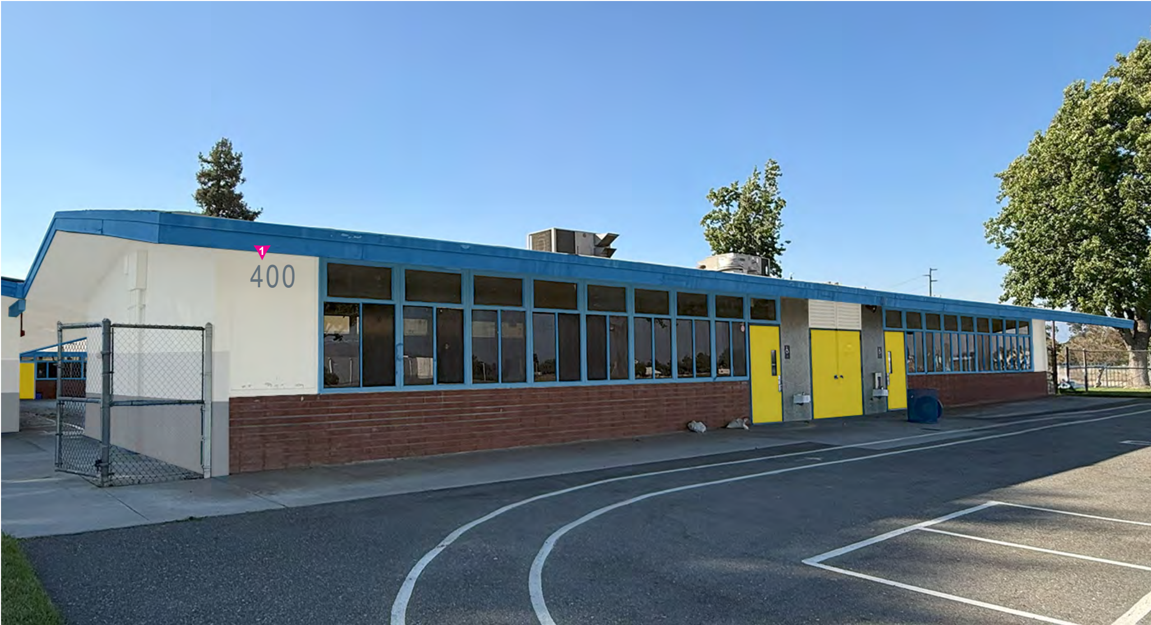
Bldg. 400 - Kindergarden CR (South Wall / North View)
