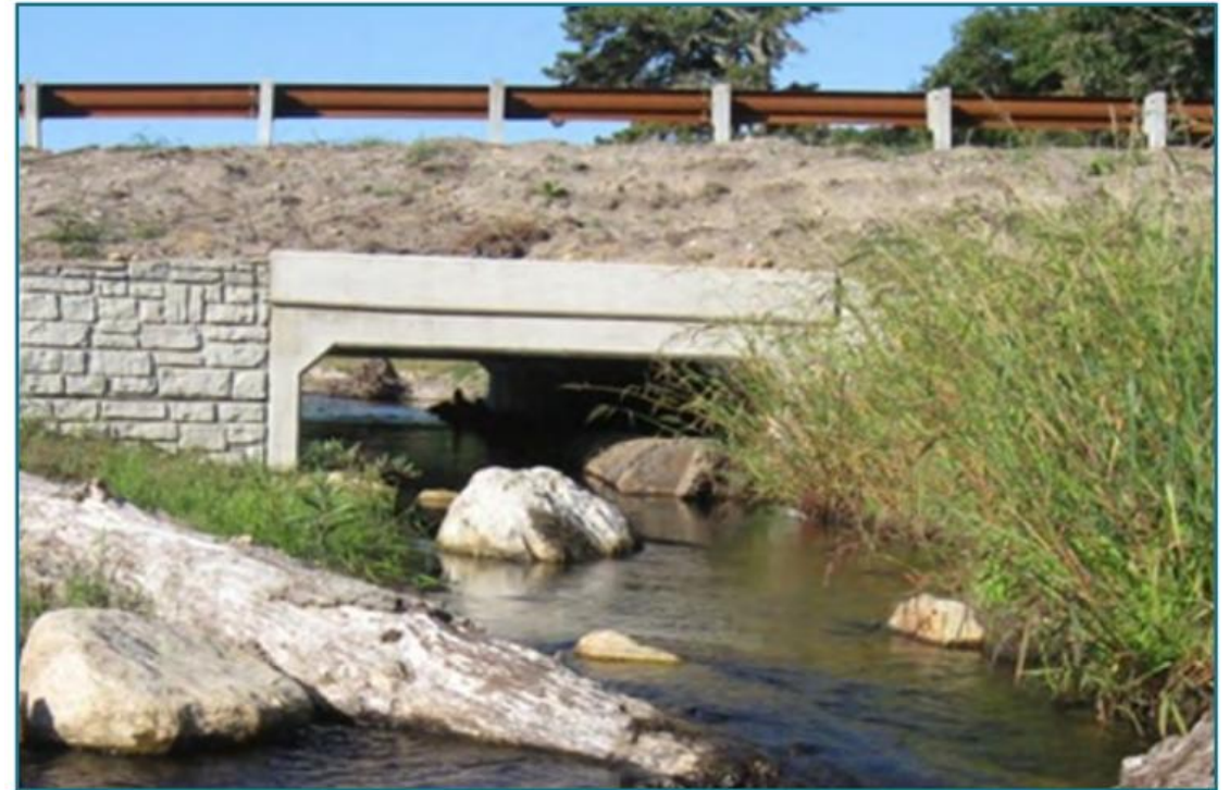
FIGURE B.4 - A reinforced concrete box structure with prefabricated wingwalls and an installed channel bed. Structure size in this example was five feet rise by ten feet span. Eel River, Plymouth, MA. Image source: Inter-Fluve.
