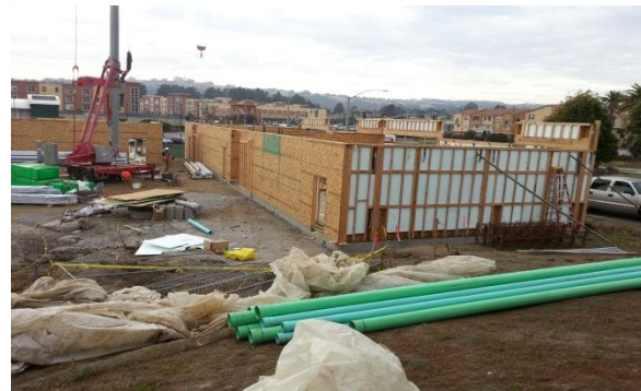
El Camino High School Science Building - January 2014
