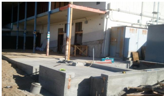
Spruce Ramp Construction – December 2013
