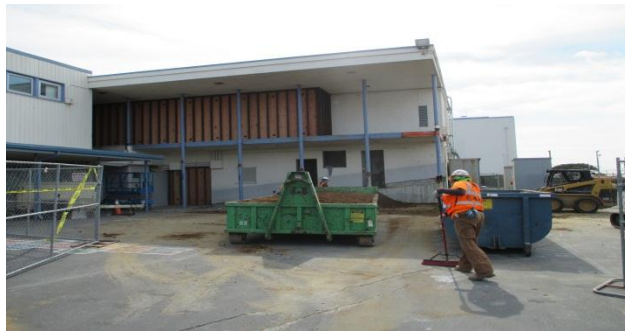
Spruce Ramp Demo – July 22, 2013
