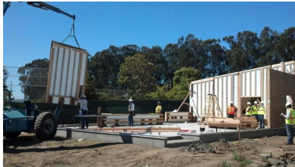
Modular Wall Installation – Alta Loma Middle School
