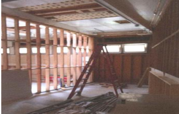
Westborough Science Framing - August 2014
