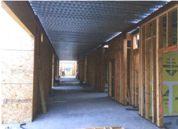
Parkway Heights Building D First Floor - October 2014
