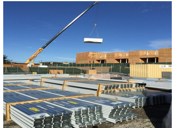
Installation of Restroom Pod – Parkway – November 2014
