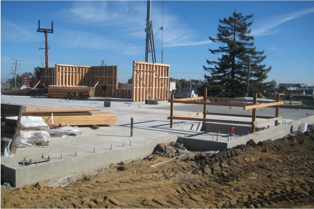
SSFHS 12 PK TWO STORY BUILDING – OCTOBER 2014
