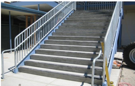
Spruce ES Staircase – May 2014
