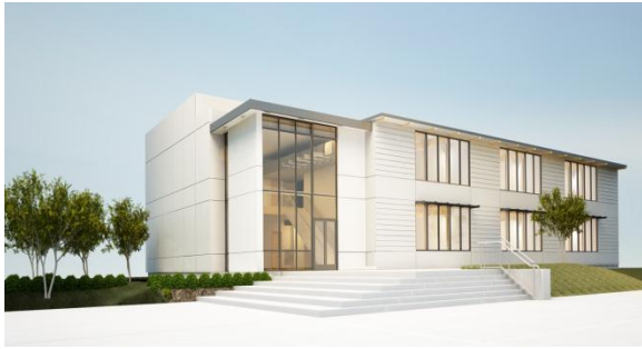
Two-story 20 Classrooms – SSFHS
