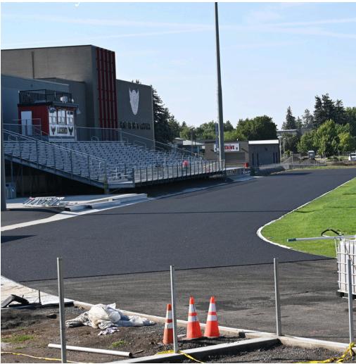
Cheney High School stadium renovation progress on July 23.
