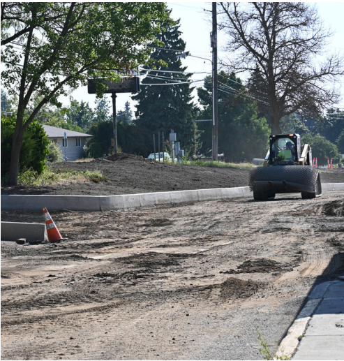
Progress on the Salnave Elementary bus loop, July 23.
