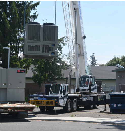
Chiller installation at Betz Elementary on June 24.
