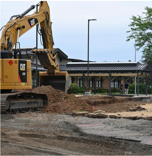
Progress on the Windsor Elementary bus loop, July 22.
