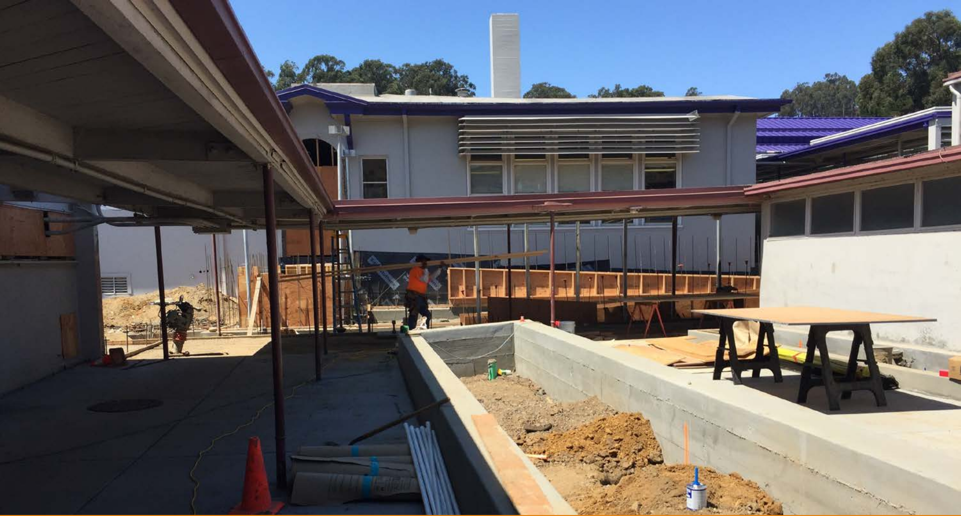
Martin Construction: Sitework new landscape planters and paving at classroom wings
