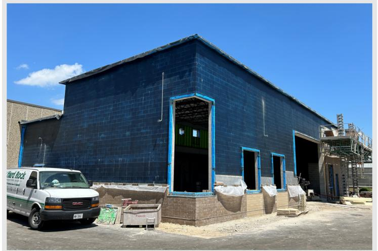
Findorff masonry crews working around the Skills Lab Addition installing brick veneer and cast stone units. Looking sharp!
