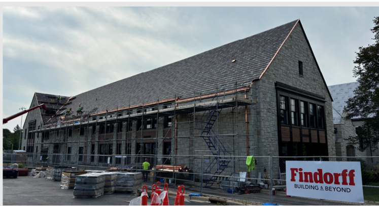
The north roof copper and LudoSlate is complete!
