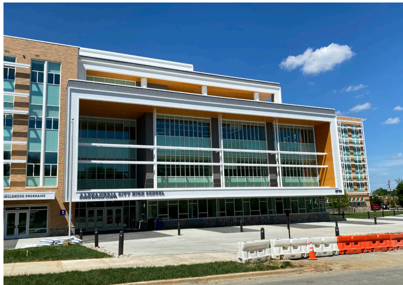
Photo 1: Exterior of Minnie Howard Near Completion
