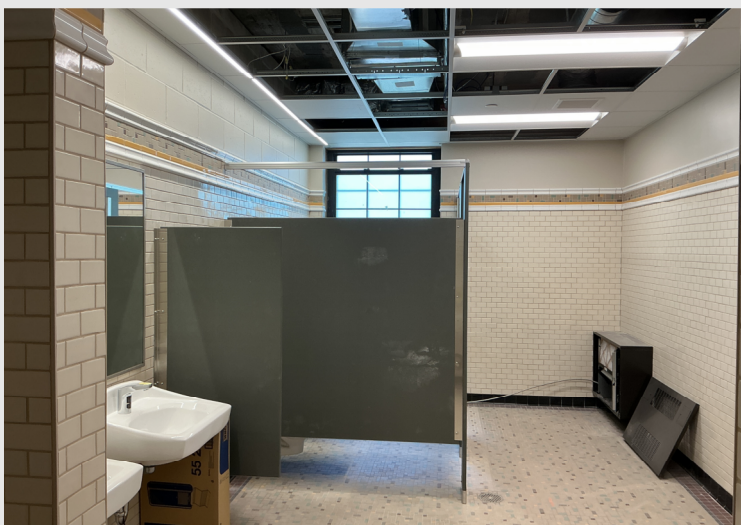
With toilet partitions installed, there are only a few remaining finishes to install to complete the Second Floor Boys Restroom!
