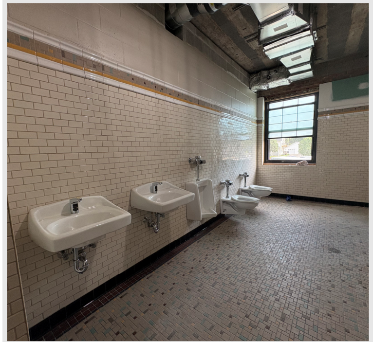
Ceramic tile is complete in the Second Floor Restrooms. New plumbing fixtures are going in place ahead of toilet partitions and accessories.
