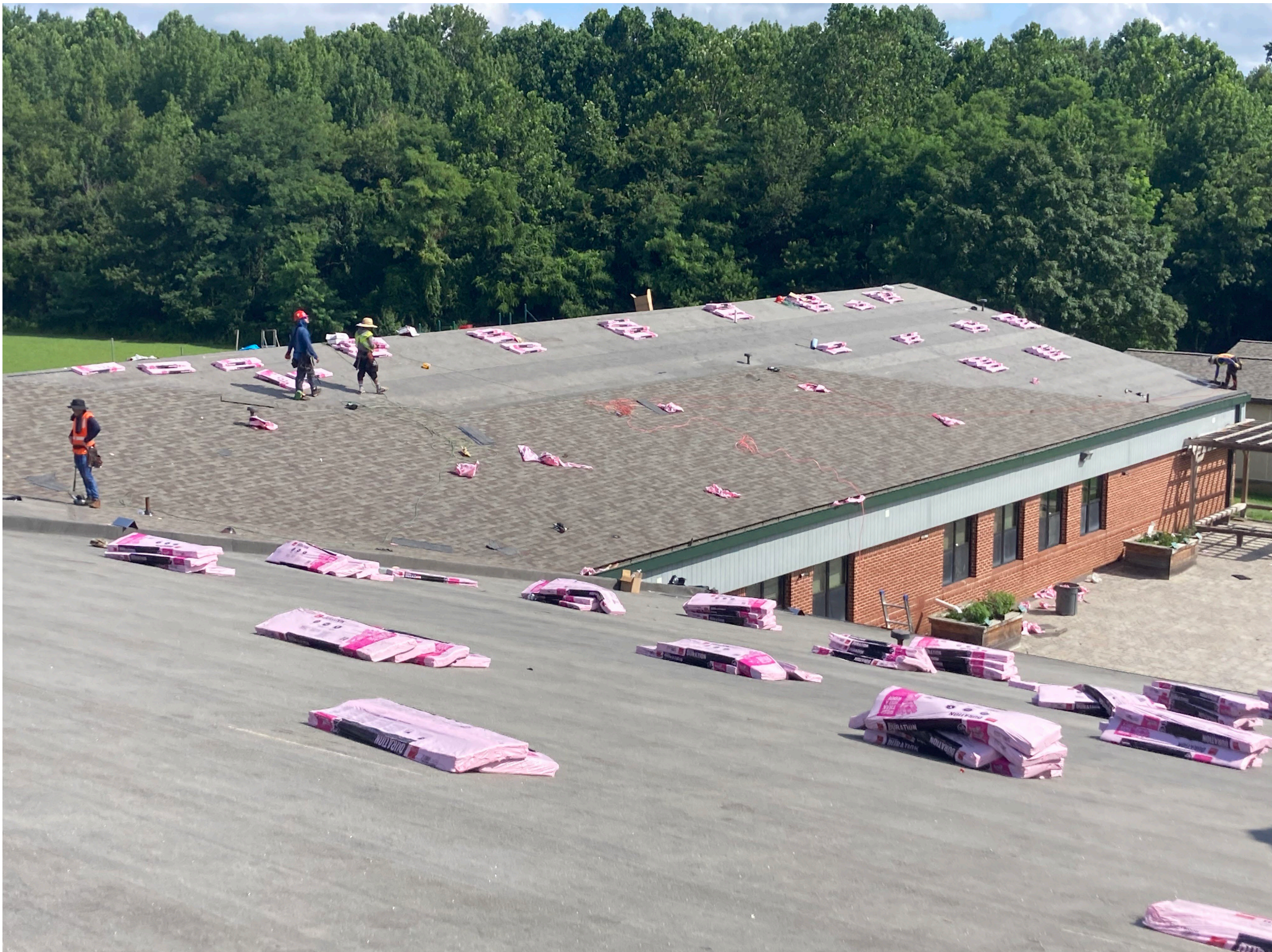
ELK NECK ELEMENTARY SCHOOL – ROOF REPLACEMENT
