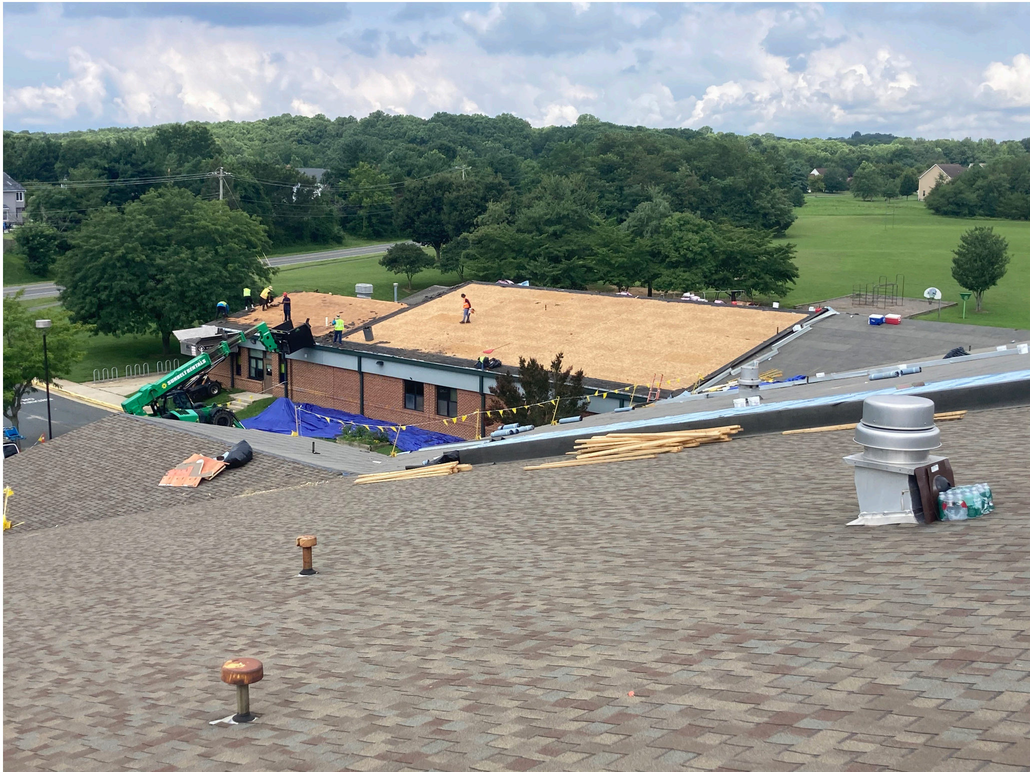
ELK NECK ELEMENTARY SCHOOL – ROOF REPLACEMENT
