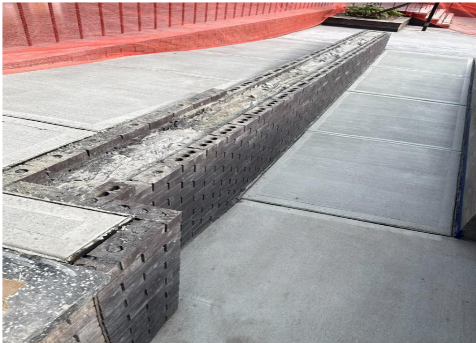
Hempstead HS – Interior Ramp
