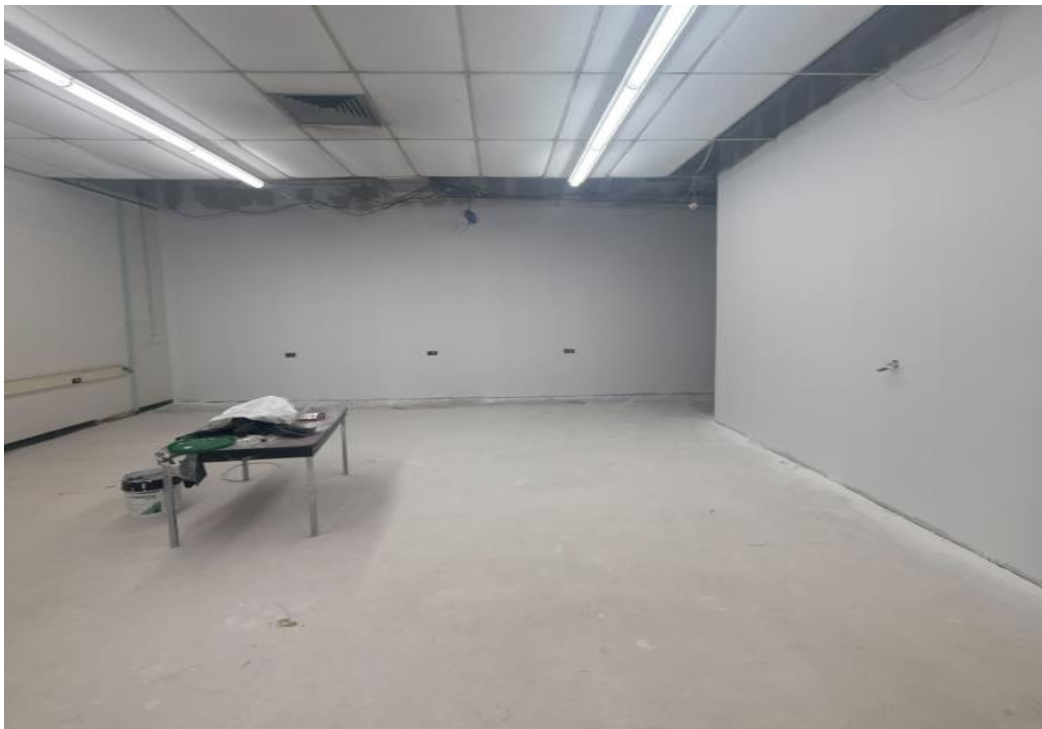
Hempstead HS – C Building Classrooms
