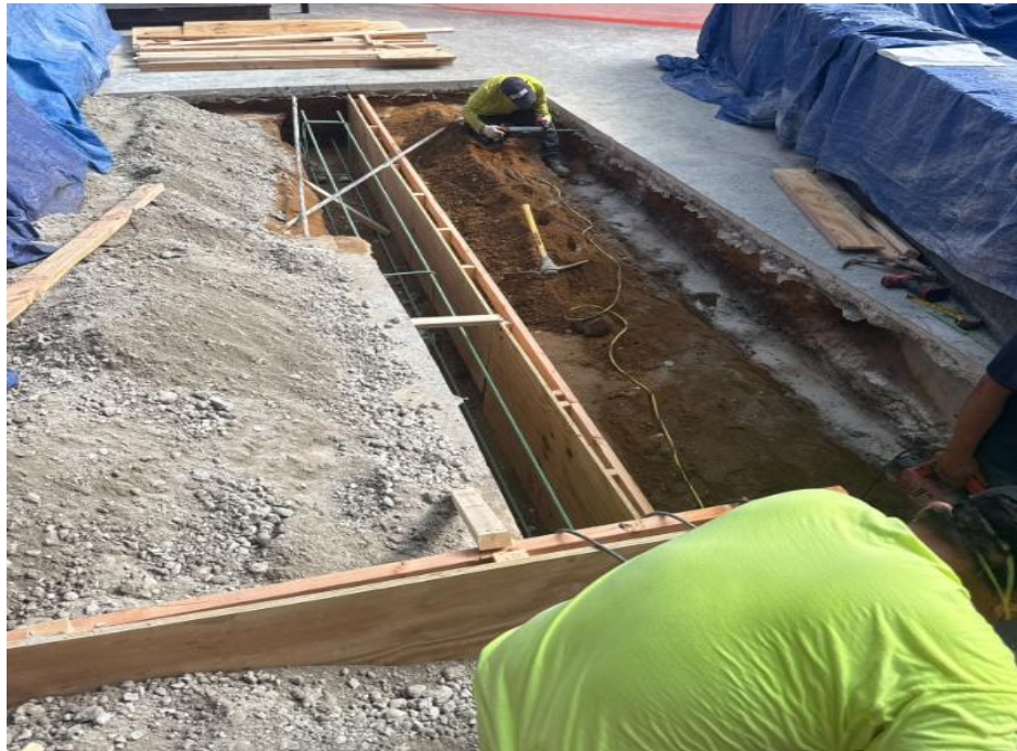
Hempstead HS – Interior Ramp
