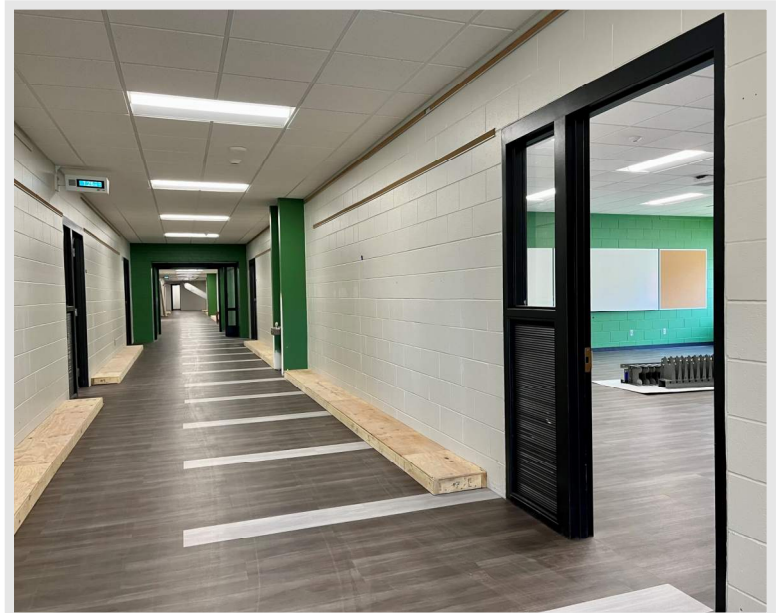
Above: a photo of the corridor finishes at Fox Prairie Elementary following installation of the new LVT flooring
