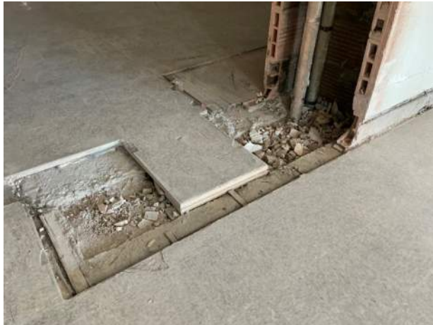
Another floor condition post demolition at the chase wall in DDC area – needing subfloor repair – between rooms 111 and 112
