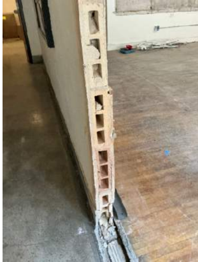
Clay tile wall at new door to Classroom 115 – will need trim to close off standard door frame depth, similar to other doors on hall with wood trim
