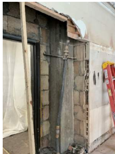
Existing condition chase wall at door demo
