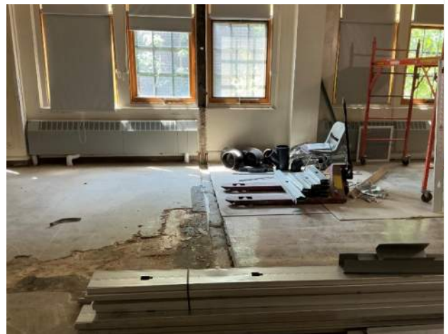
DDC area floor - existing conditions to be modified so flooring can go down – and up exterior wall at removed interior wall will need patching
