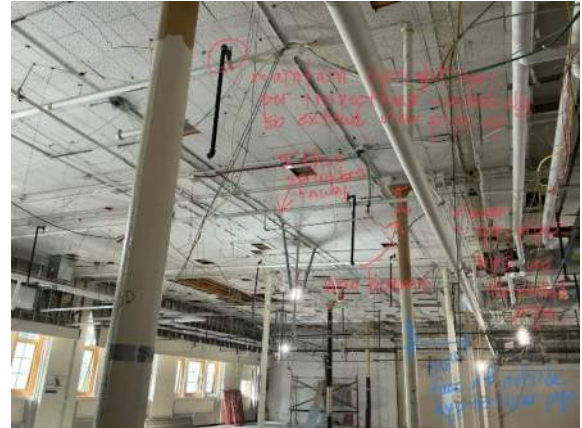
Reviewed sprinkler piping that was above drop ceiling that conflicts with new steel beams, will need to be revised
