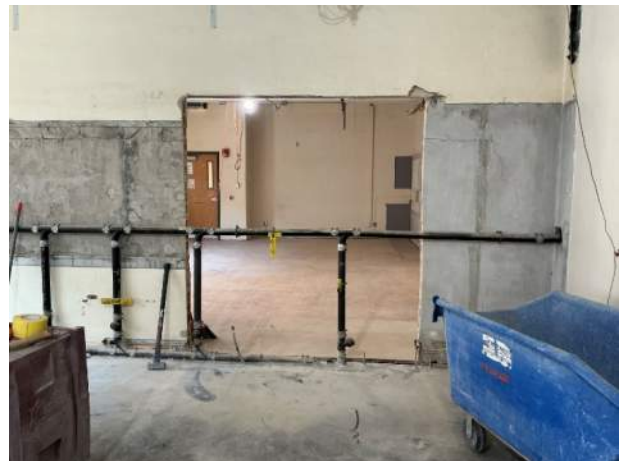
Larger view of new door opening to storage – also to left uneven wall from chalkboard abatement
