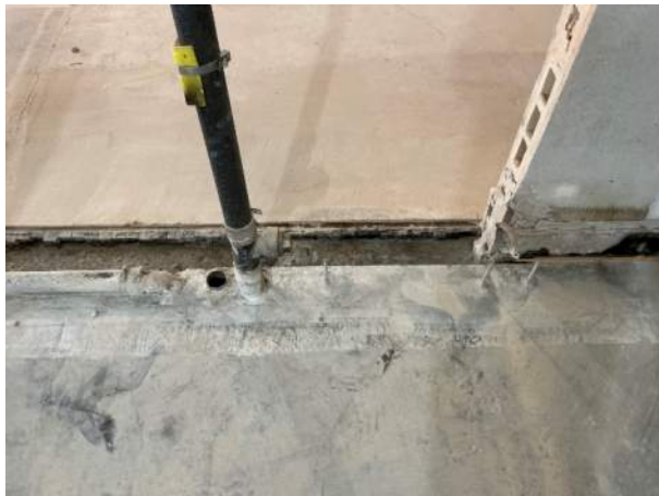
New door opening to storage – floor poured either side to wall so will need to address door threshold area
