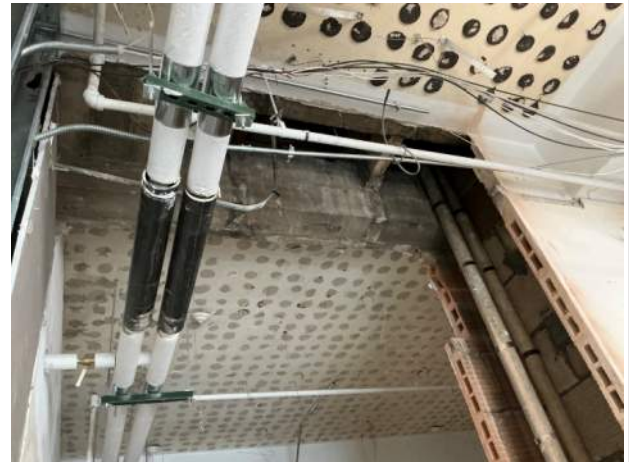
Room 111 opening at chase wall head condition
