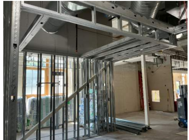
Framing including ceiling soffit at new CTE entry
