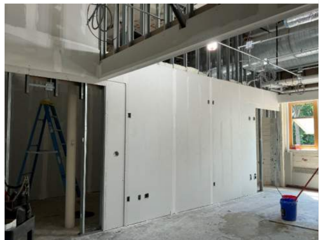
Gypsum board installation
