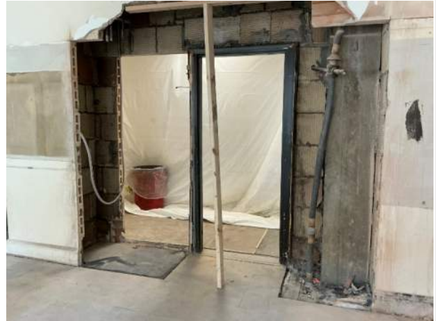
Scene shop new door opening and existing conditions to address within the chase space
