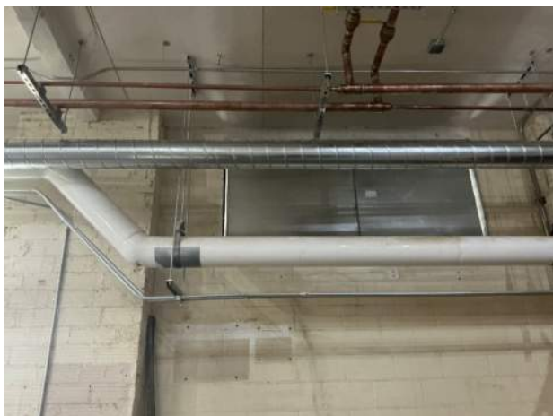
Construction Lab infill at removed mechanical
