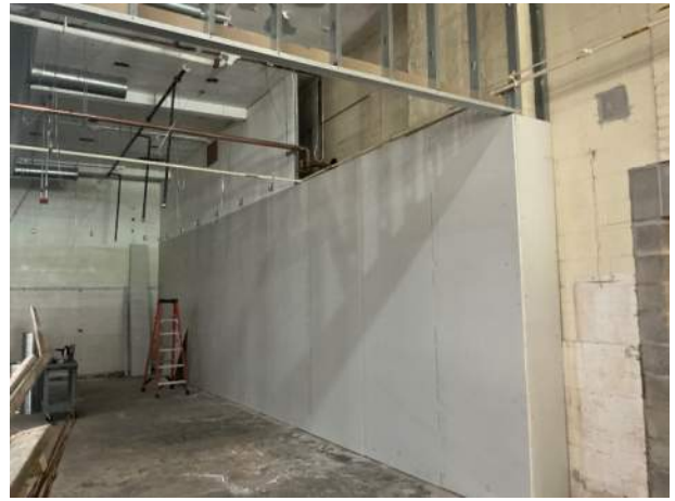
Construction classroom wall with gypsum board
