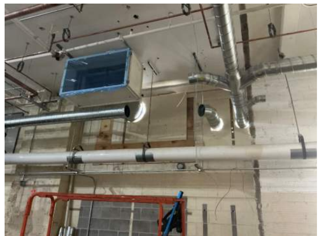
Dust collector ductwork entry from exterior status
