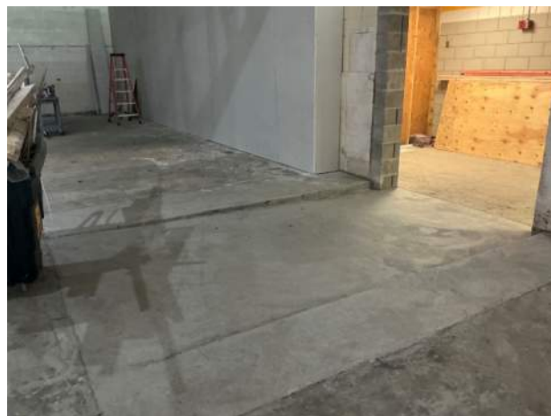
Construction Lab ramp poured
