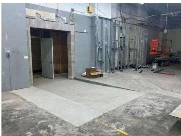
Collision Lab ramp poured
