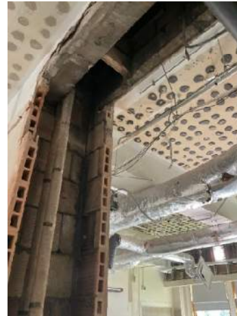
Room 111 opening at chase wall head condition – reviewed this week that existing pipes go multiple floors so needed shaft construction detail – see PR 20
