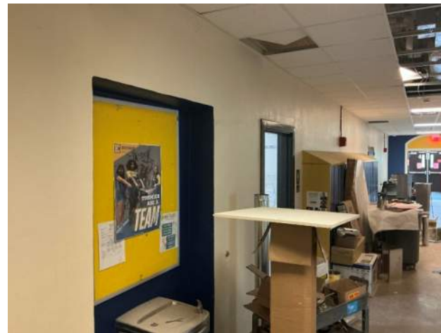
DCD bath room review existing conditions for PR – demolition of the wall as indicated in CD's would require more rebuild including ACT ceiling than anticipated and than schedule allows
