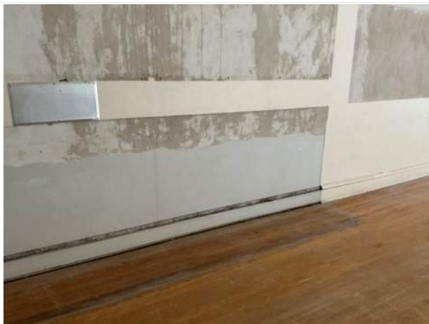
More patch areas for PR 17 – Storage 105E was closed off for abatement at the time and now visible – this is also for the wood base – missing shoe and cap.
