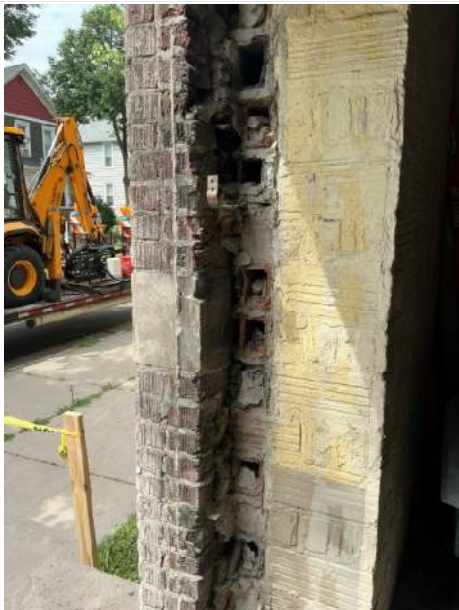
Exterior entry wall construction with all layers
