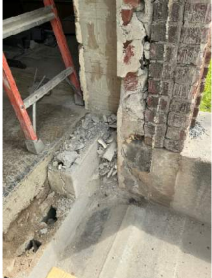
Exterior entry wall section – 2 layers brick and 2 layers backup - unexpected
