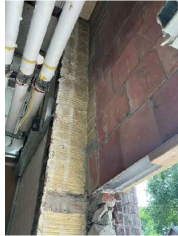
Exterior entry wall above door level- lintel at door not resting on backup wall structure fully – take all down
