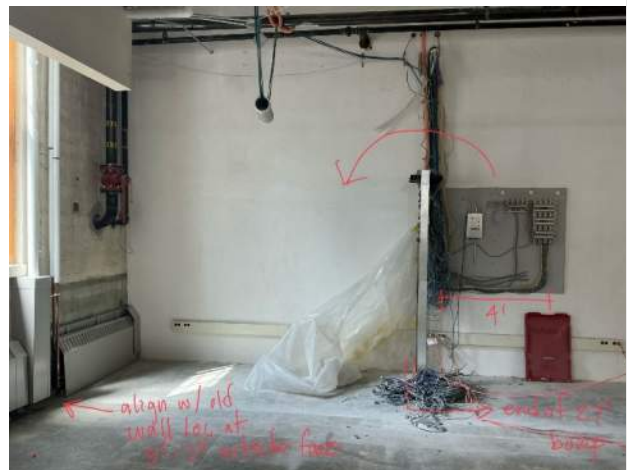
Gas closet area to be enlarged to enclose the remaining data as shown and in PR 19.
