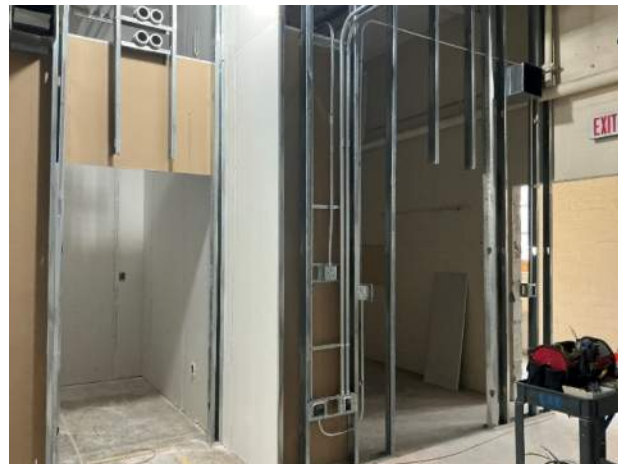
Office and data room framing and gypsum board
