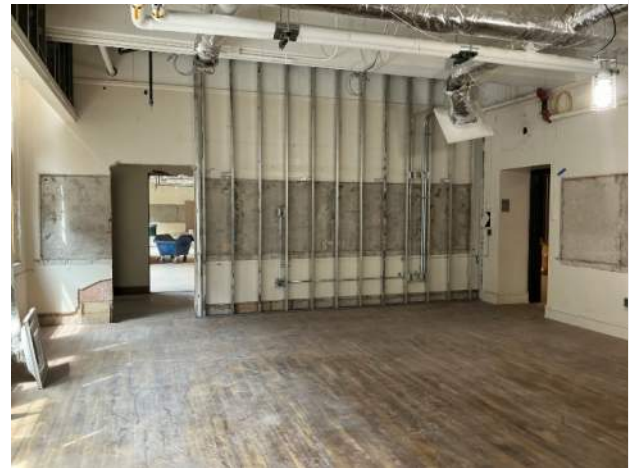
Framing at Room 115 and patch to left- reviewed on site to continue framing to corner
