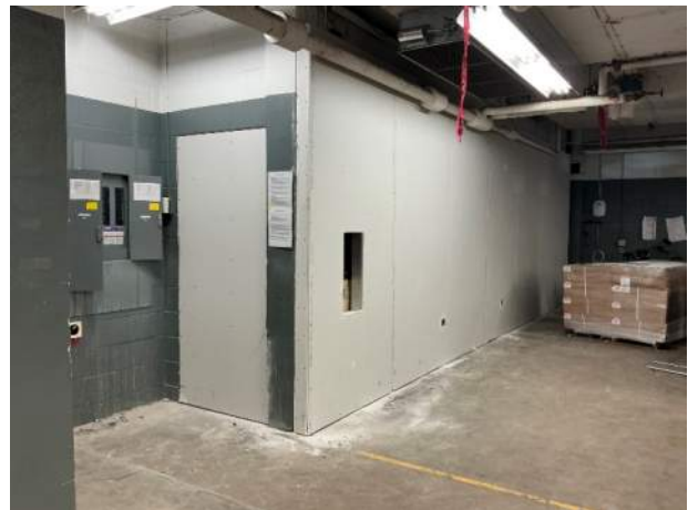
Temporary wall from Auto Repair side with gypsum board installed
