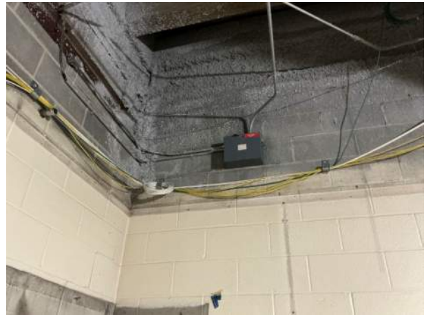
Traced conduit to the controller for Door 13
