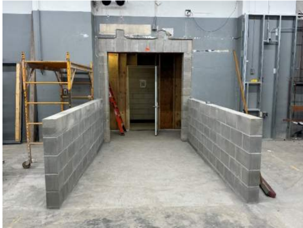
Collision Lab ramp with masonry installed
