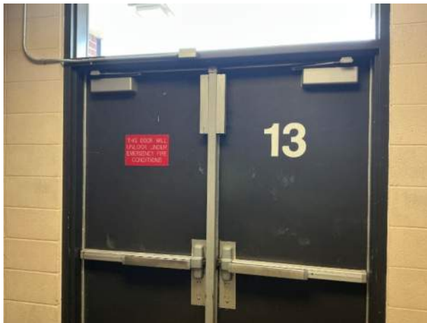
Door 13 mag locks in place – cannot verify operational as building in test mode
