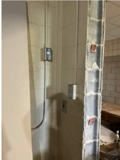
Reviewed existing conditions for Door 13 hardware – key switch in place in Admin room
