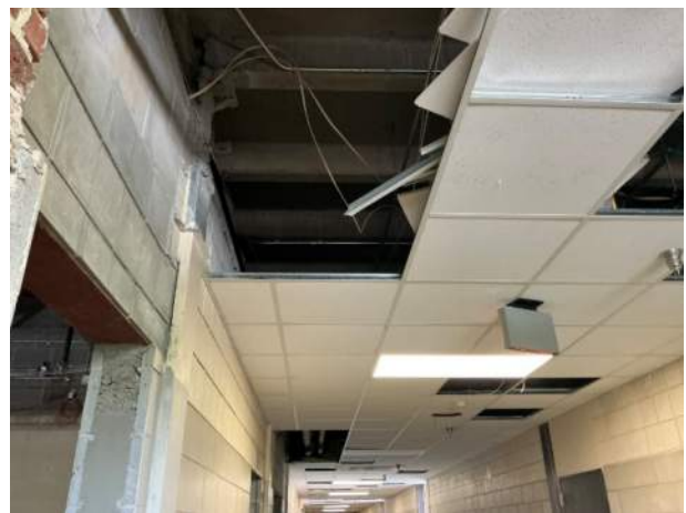
Hall at admin end showing existing structure for wall framing above new storefront
