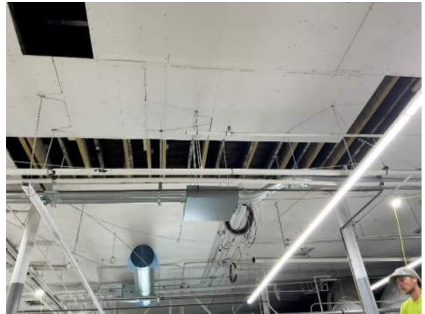
Collision Lab structural LVL installation
