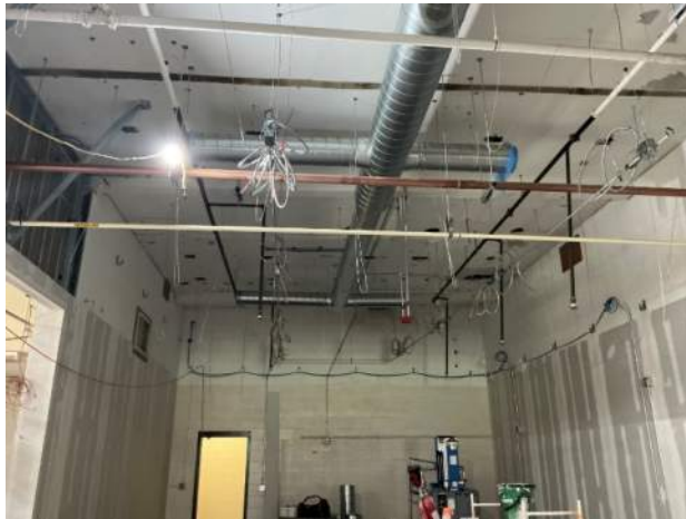
Construction classroom taped at gypsum board and MEP installation
