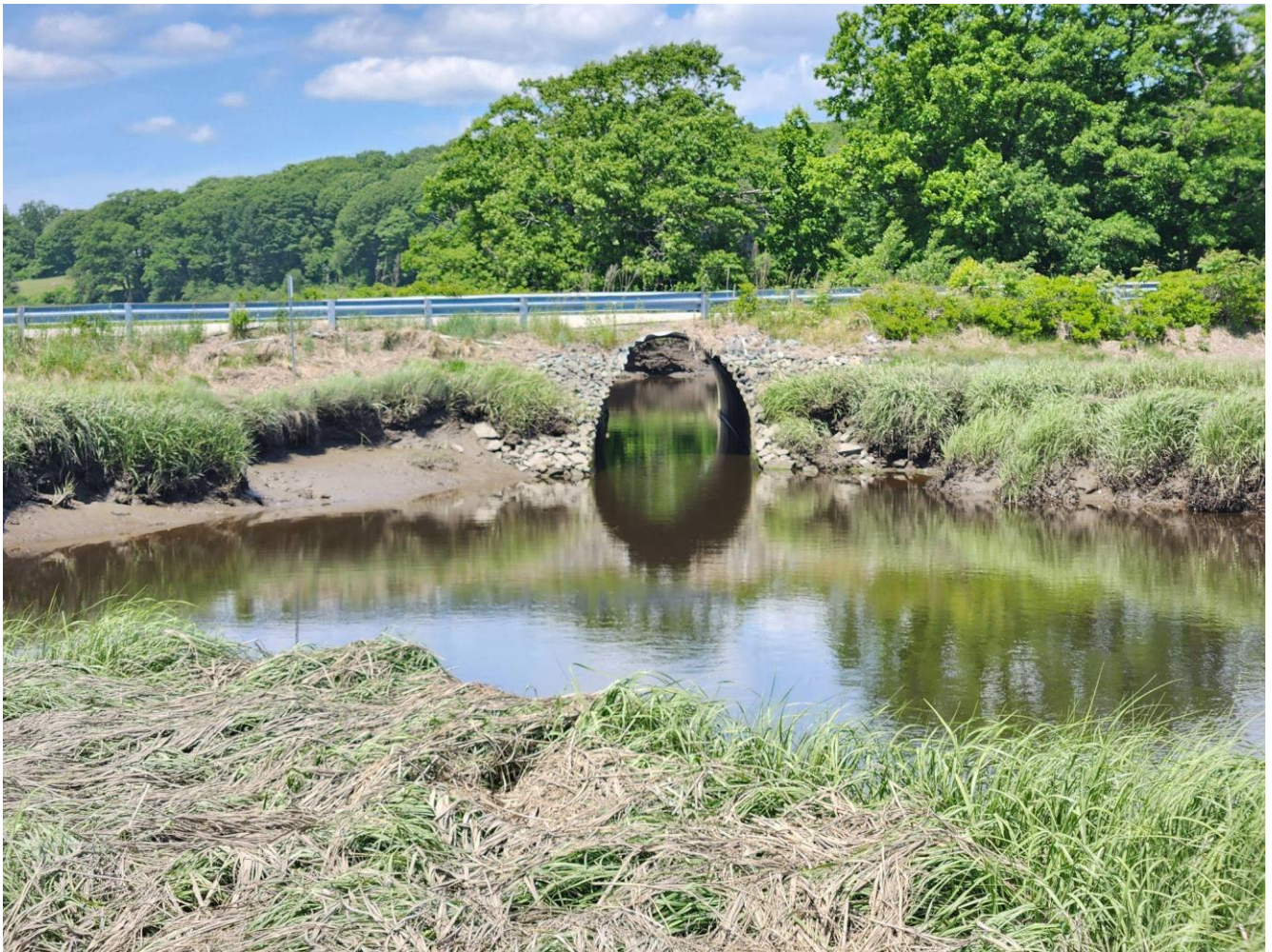
Figure 2. The tidal culvert under Sawyer St/Rd restricts tidal flow, as evidenced by the large scour pools and eroded marsh banks adjacent to the crossing (WNERR, 2024).
