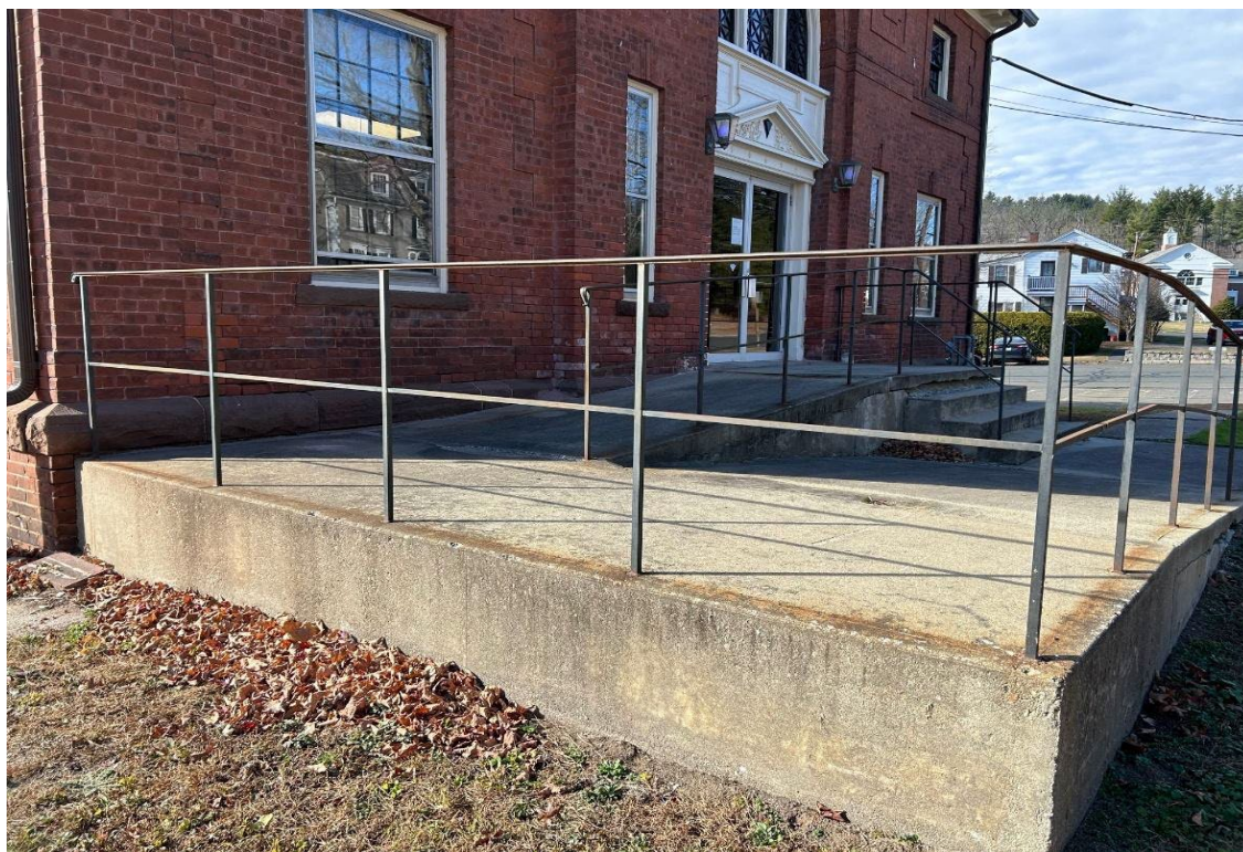
Side view of ramp
