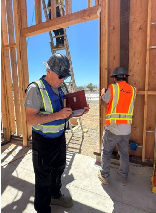
Structural Testing, everything is tested.
