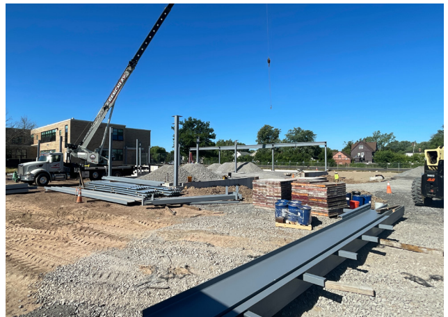
Steel beam installation for new UPK addition at Windermere Boulevard Elementary School
