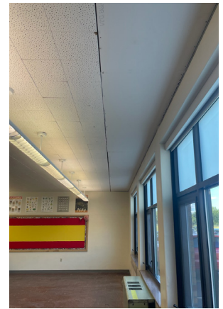
Amherst Middle School classroom improvements
