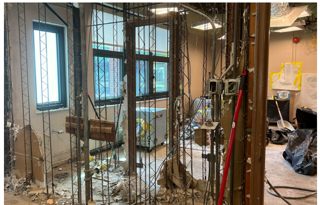
Demolition of the main office space at Smallwood Drive Elementary School
