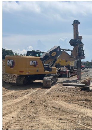
Installation of lighting foundation at new athletic turf field
