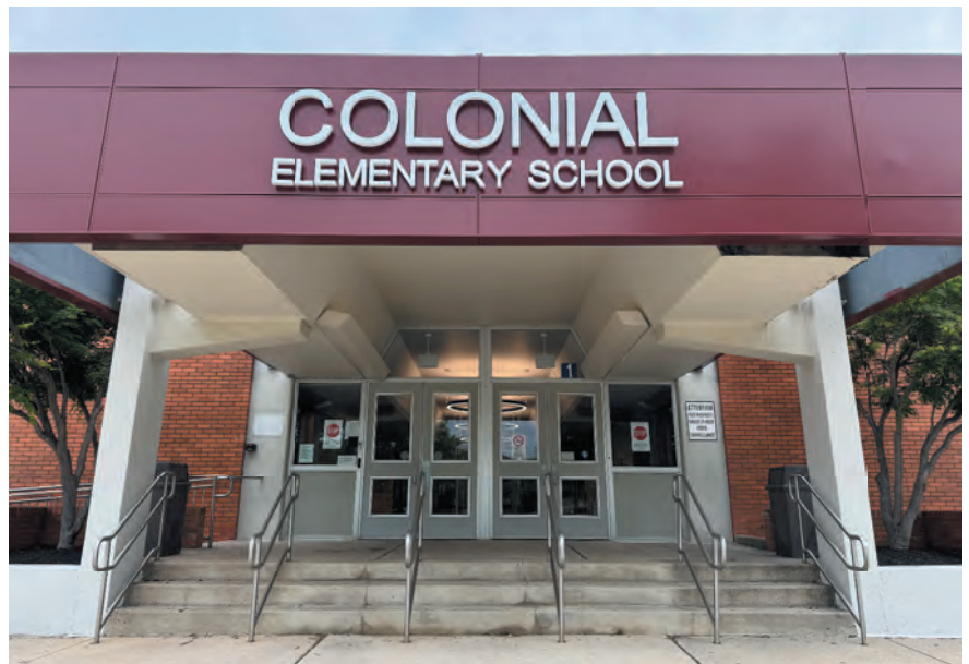
Part of the renovation project included new signage to clearly indicate the main entrance for the school.
