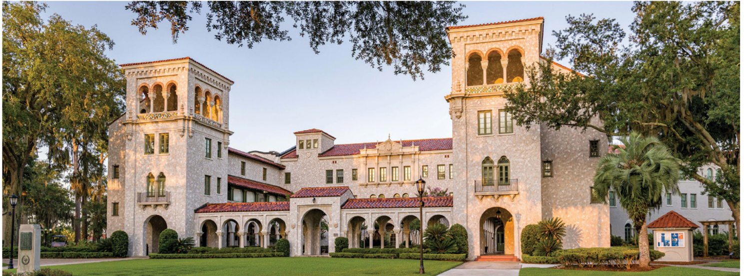
Renovations are underway to transform classrooms and staff offices of the former hotel building at The Bolles Upper School San Jose Campus into dorms, common and support areas and dorm parent apartments.
