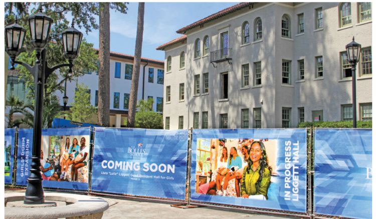
Work has begun for phase II of The Bolles School's Llura "Lulie" Gund '58 Residence Hall for Girls.
