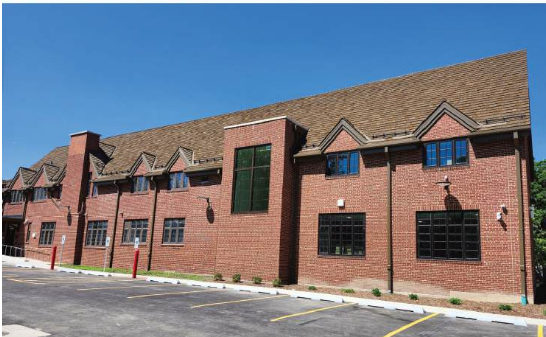
The new main stairway and elevator and stairs addition as seen on the right in the rear of the school. The brick and gable elements were made to match Irving Pond's work.
