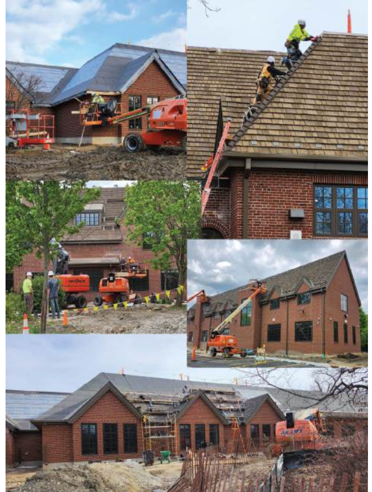
Ravinia School construction scenes, December, 2024 - June, 2025 Photo by Elliott Miller
