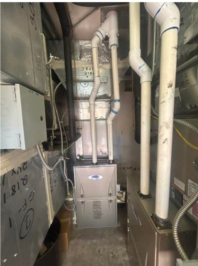
IMG_9096 KFI Engineers May 6, 2025 2:32 PM
