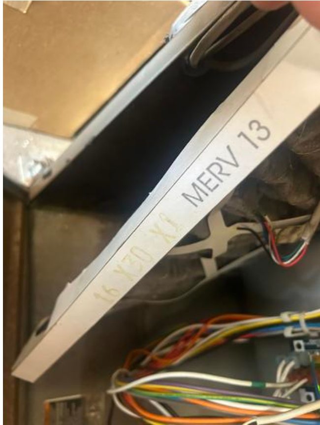
IMG_9102 KFI Engineers May 6, 2025 2:32 PM
