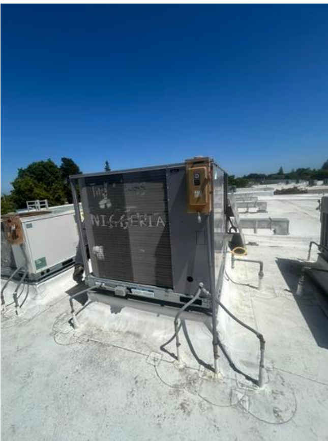
IMG_9129 KFI Engineers May 6, 2025 3:23 PM
