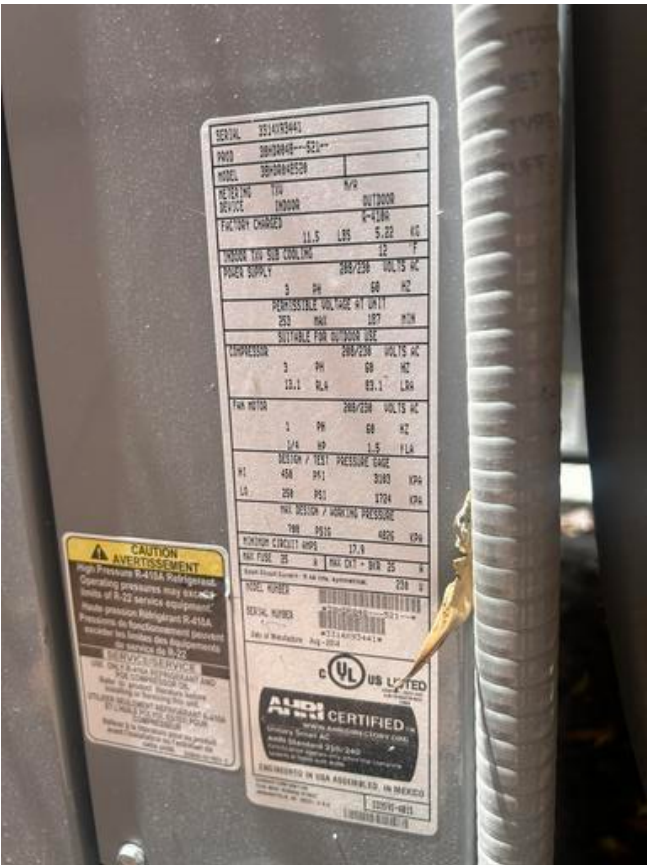
IMG_9120 KFI Engineers May 6, 2025 2:39 PM
