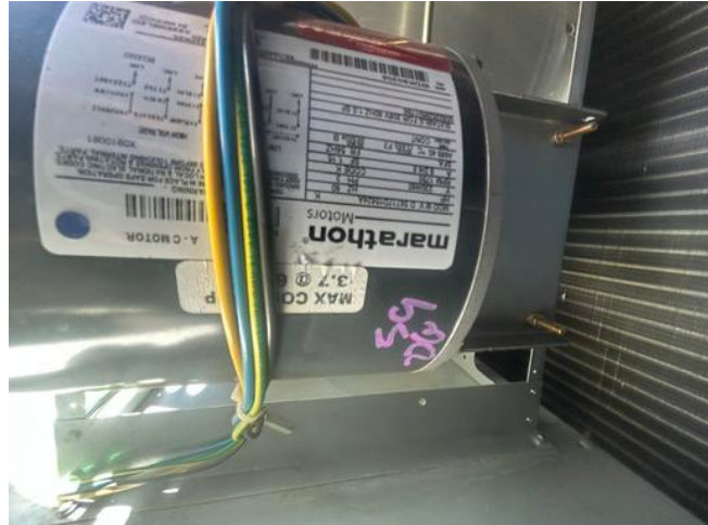
IMG_9132 KFI Engineers May 6, 2025 3:23 PM
