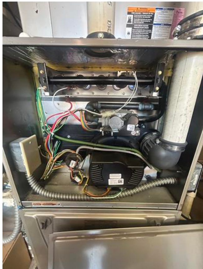
IMG_9100 KFI Engineers May 6, 2025 2:32 PM
