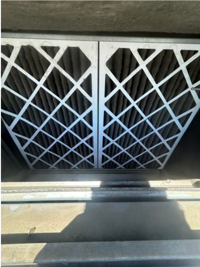
IMG_9143 KFI Engineers May 6, 2025 3:26 PM
