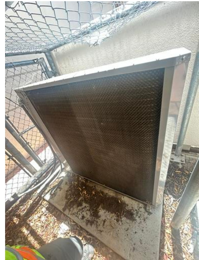
IMG_9119 KFI Engineers May 6, 2025 2:39 PM
