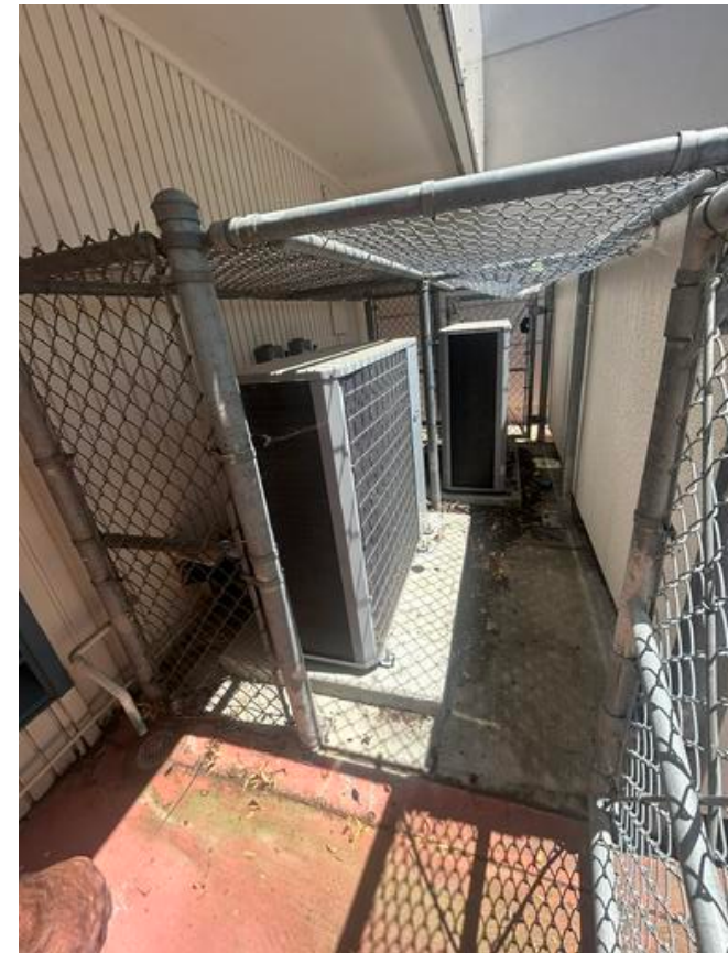
IMG_9116 KFI Engineers May 6, 2025 2:39 PM
