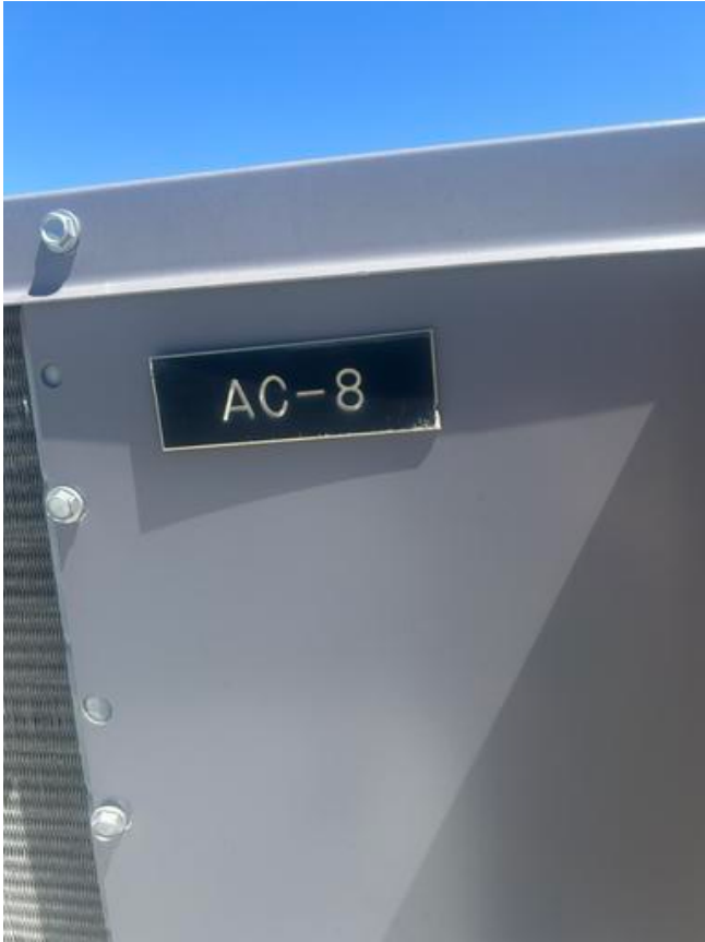
IMG_9130 KFI Engineers May 6, 2025 3:23 PM
