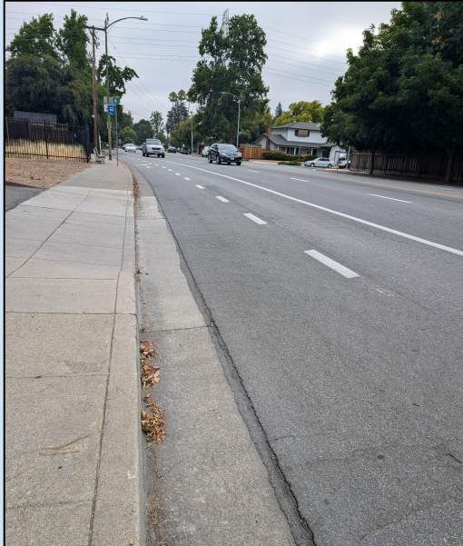
Bike lane markings faded
