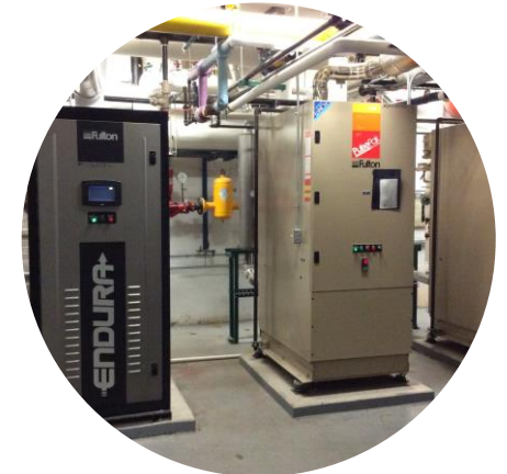
Boiler & Hot Water Replacement
