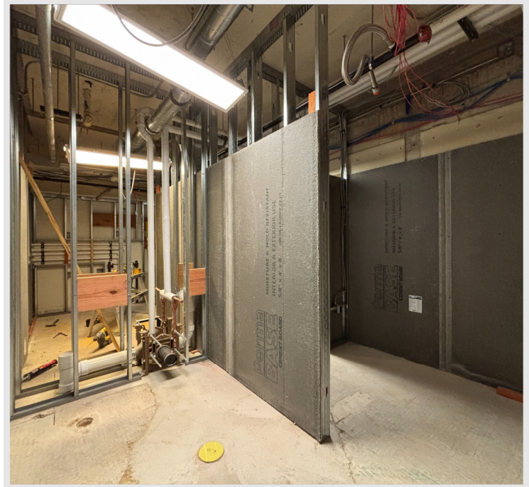
View from inside the Lower-Level Restrooms with framing complete and cement board in progress to provide substrate for ceramic tile!
