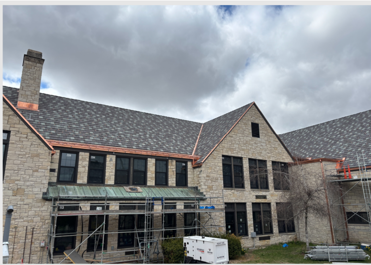
A look at the nearly complete tile work and upper metal batten roof on the west elevation of the Courtyard. The copper looks awesome!
