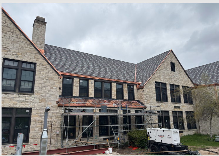
Updated look at the complete tile and upper metal batten roof on the west elevation of the Courtyard. Lower metal batten roof in progress!
