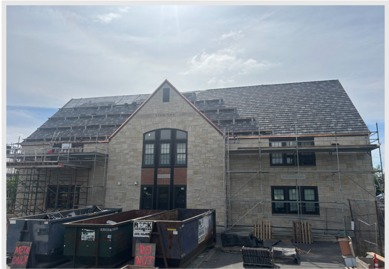
Check out the final roof installation above the Library with the sun shining and slate tile in progress. Almost wrapped up!
