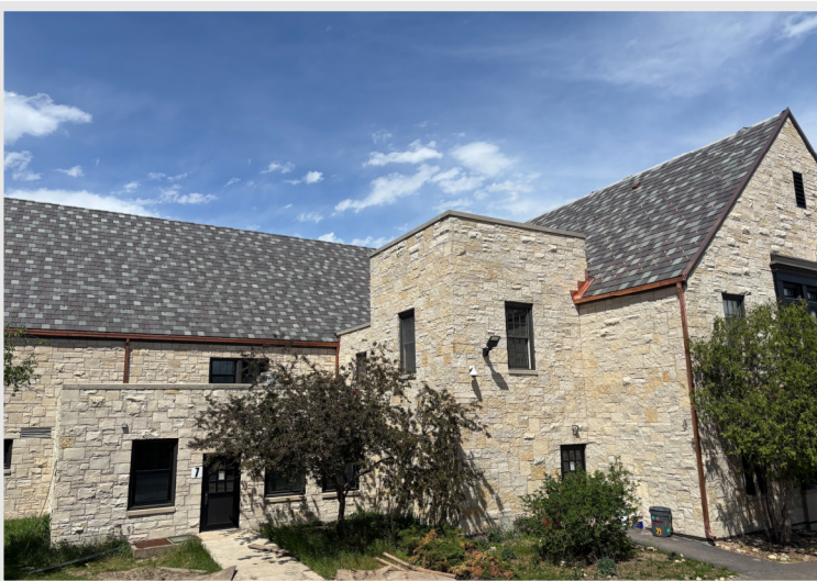
A view of the completed slate tile, sheet metal, and gutters on the roof over the courtyard's north elevation!
