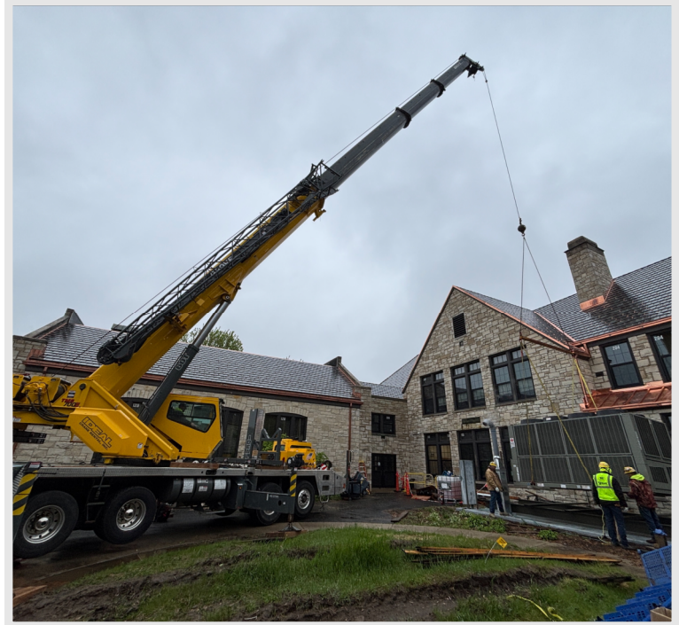
A recent view from the courtyard observing the crane pick to set the new chiller unit. Looking forward to getting this unit operational soon!
