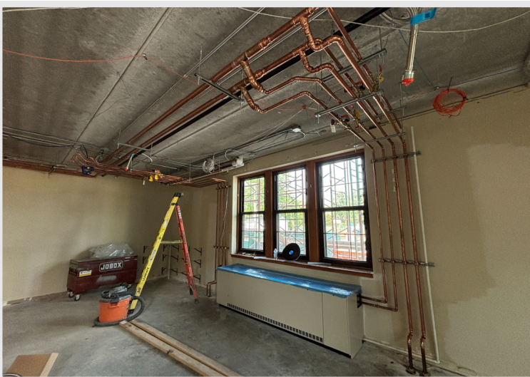
A look inside the First Floor 5K Classroom with the full mechanical piping system in place to the new unit ventilator!
