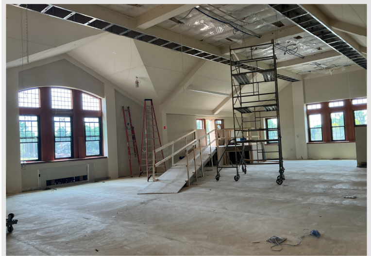
An inside look at the demolition wrapping up in the Library. These soffits will receive the new sprinkler system to bring protection into this space!
