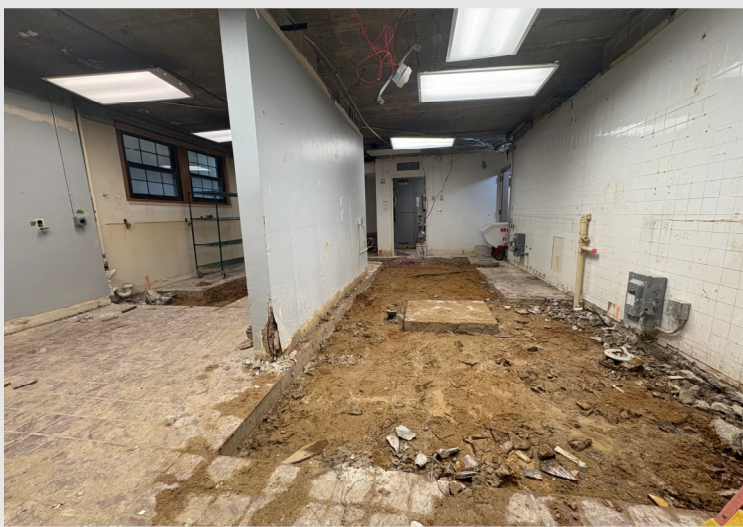
Concrete slab removal in progress in the Kitchen. New underground work will follow to upgrade the system for the space's equipment.
