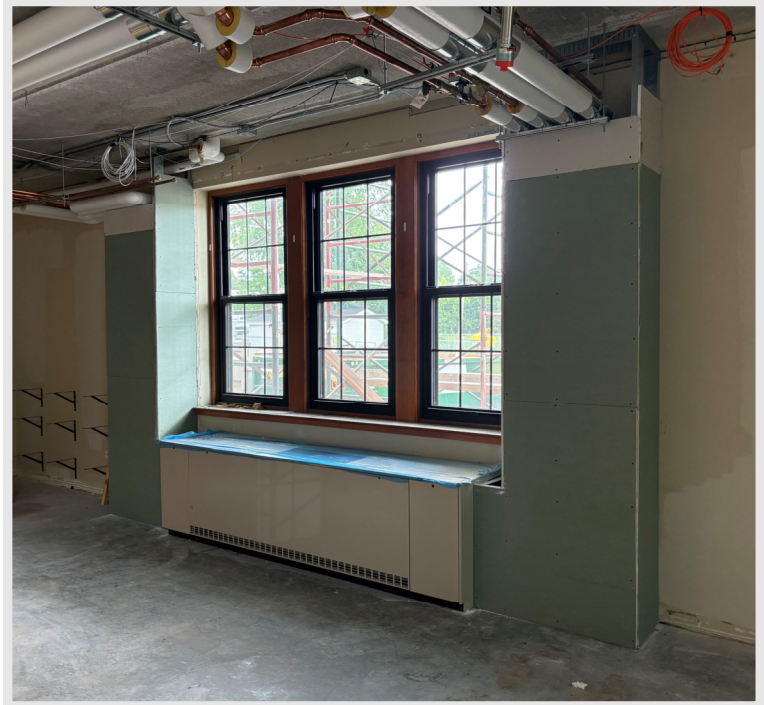
The new unit ventilator installed in the First Floor 5K Classroom with the pipe chases insulated and drywalled. Ready for finishes!
