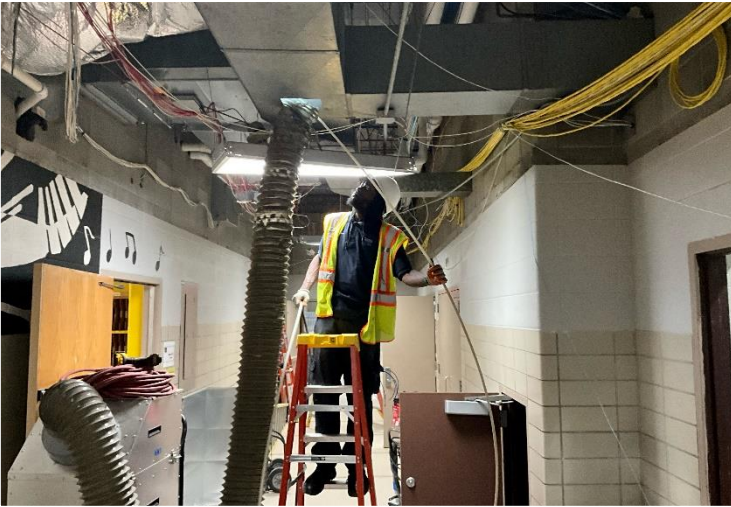
MS/HS - Area A - Duct Cleaning In Progress
