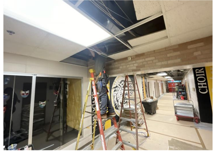
MS/HS - Area A - EC Performing Rough-Ins
