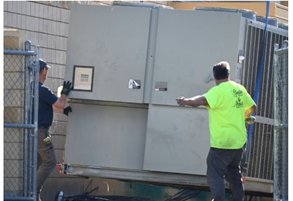
Salnave Chiller – Crane Rigging
