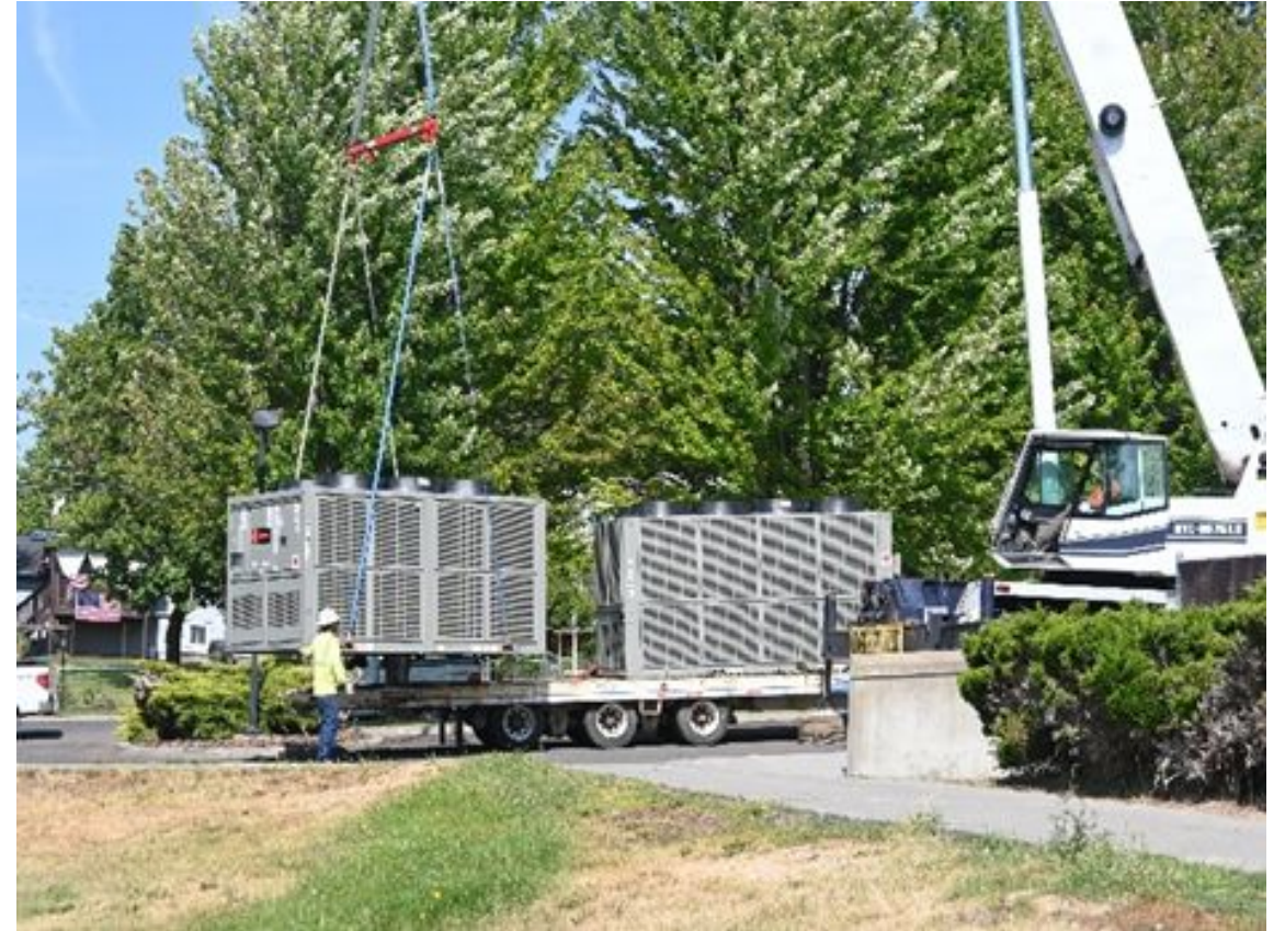
Salnave Chiller – Crane Rigging
