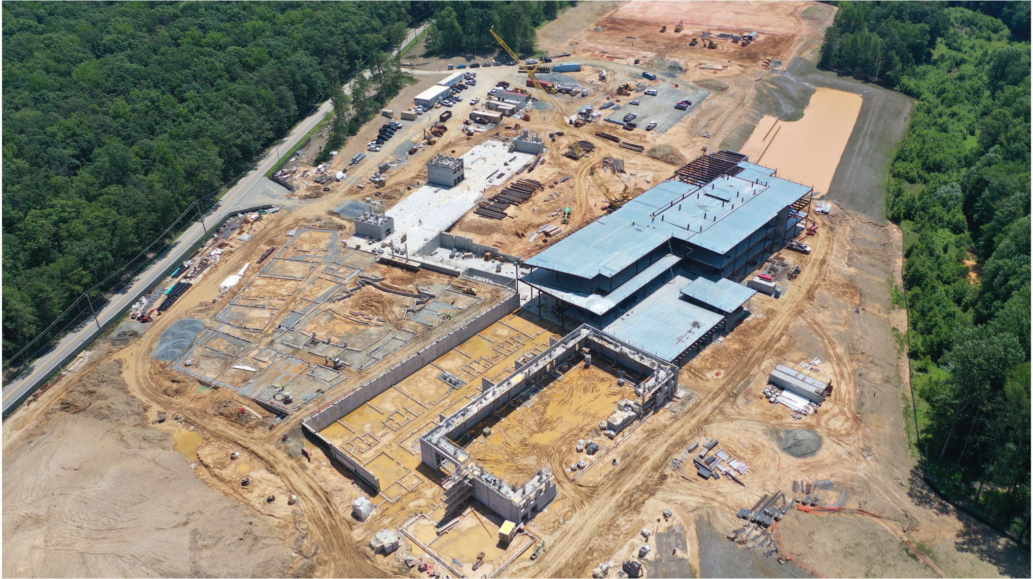
NORTH EAST MIDDLE / HIGH SCHOOL – REPLACEMENT
