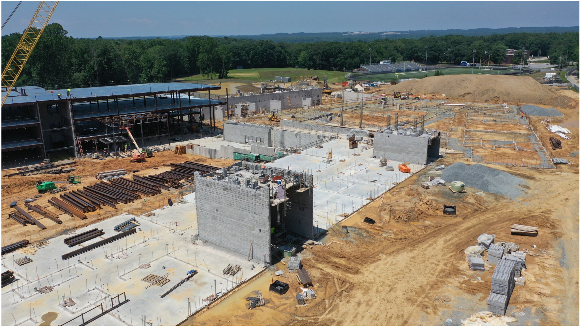
NORTH EAST MIDDLE / HIGH SCHOOL – REPLACEMENT
