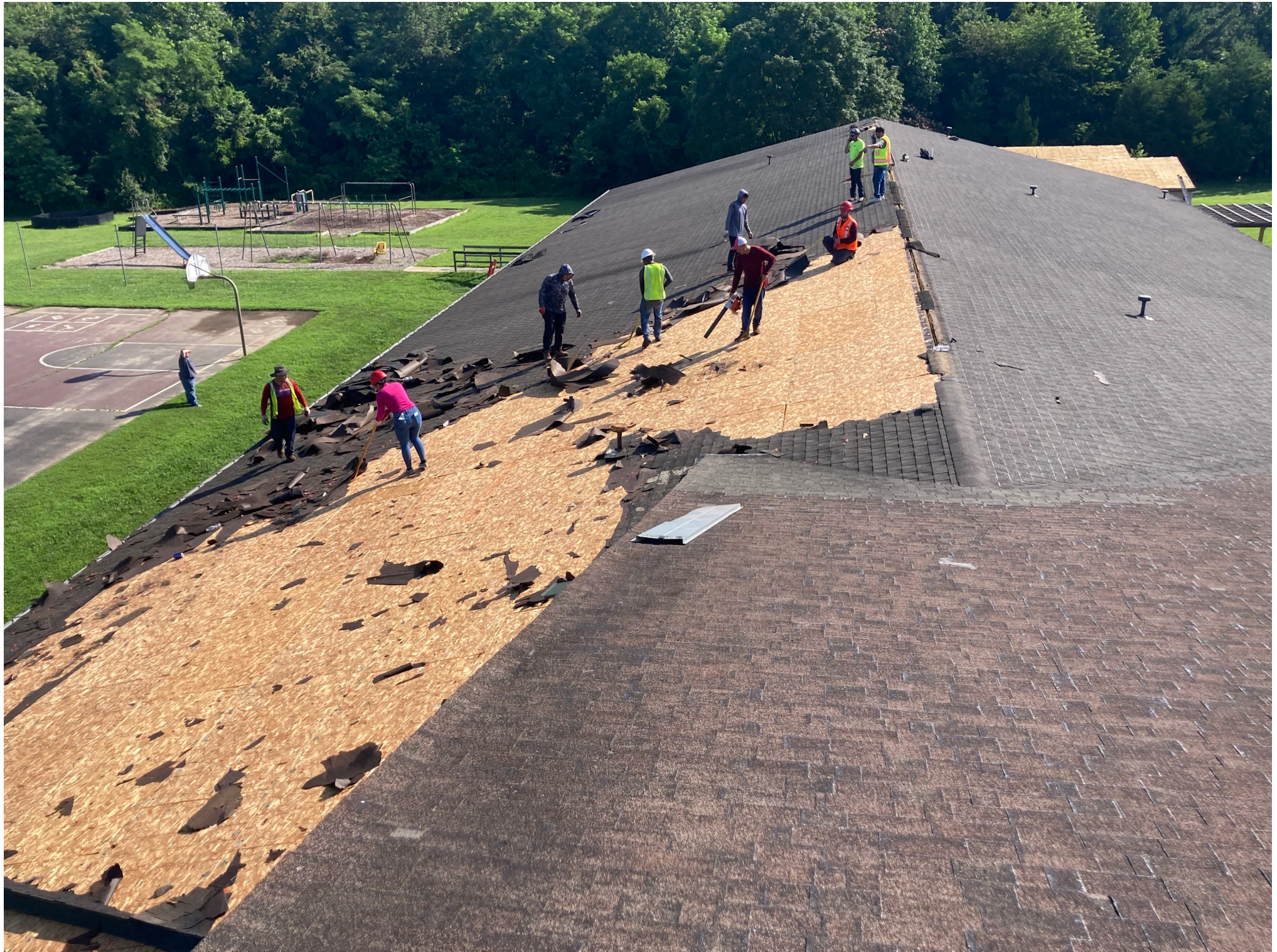
ELK NECK ELEMENTARY SCHOOL – ROOF REPLACEMENT
