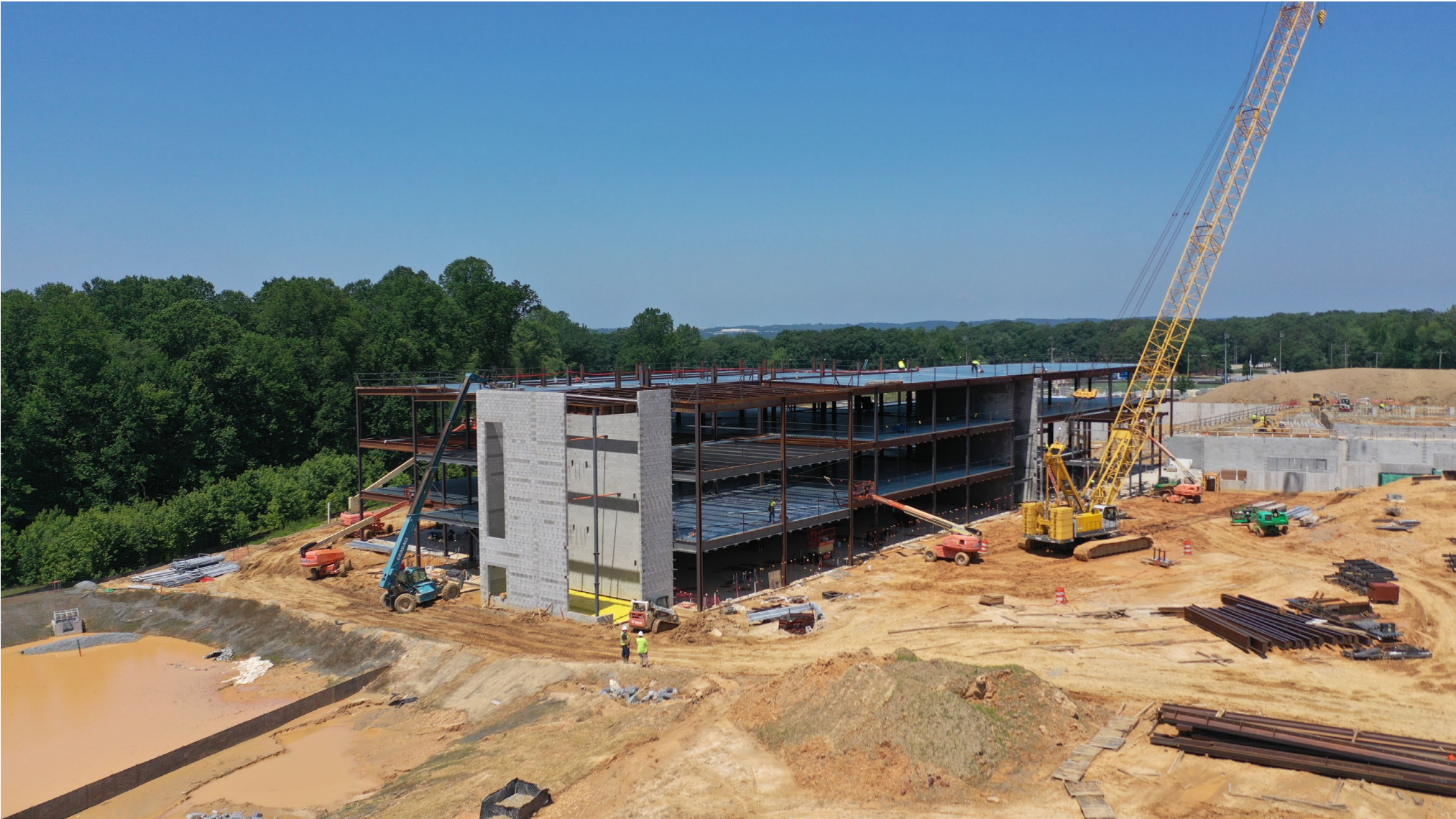
NORTH EAST MIDDLE / HIGH SCHOOL – REPLACEMENT
