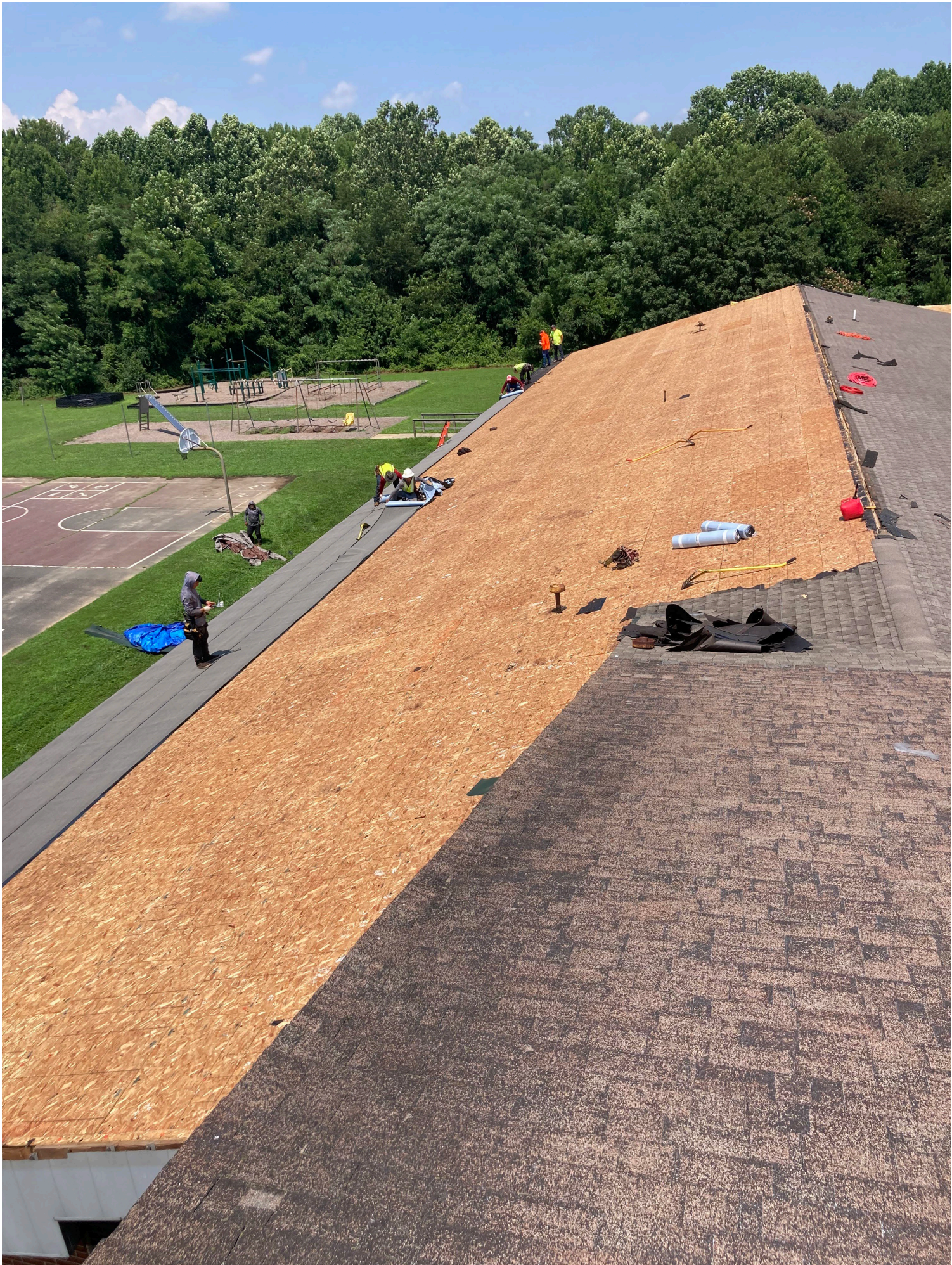
ELK NECK ELEMENTARY SCHOOL – ROOF REPLACEMENT
