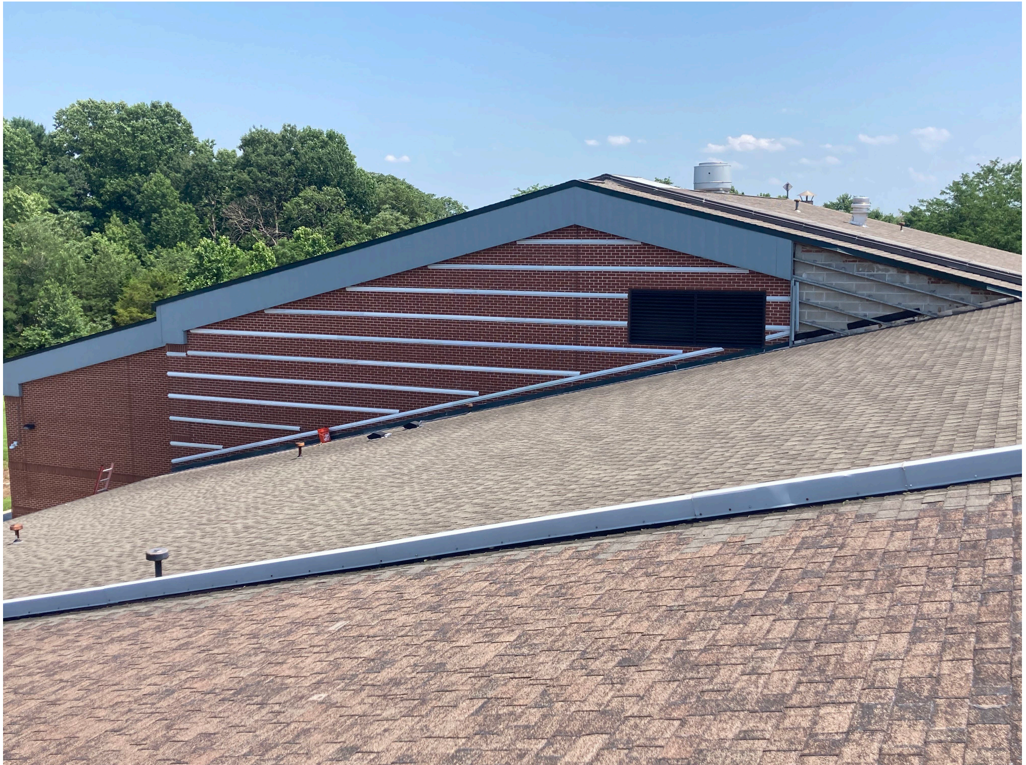
ELK NECK ELEMENTARY SCHOOL – ROOF REPLACEMENT
