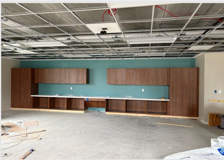
Inside the First Floor 5K Classroom with the walls recently painted, ceiling grid in place, and the new casework and countertop installed!
