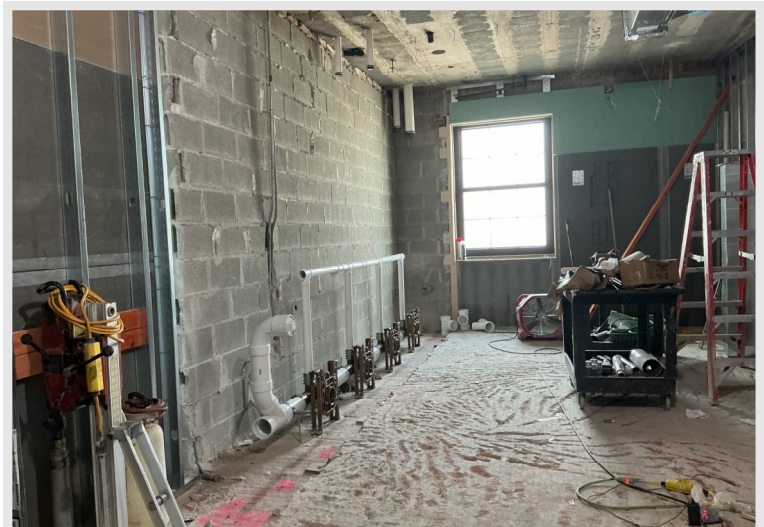
New rough-in work in progress for the First Floor Restrooms. Once complete, new block walls will be built to reshape this restroom space!
