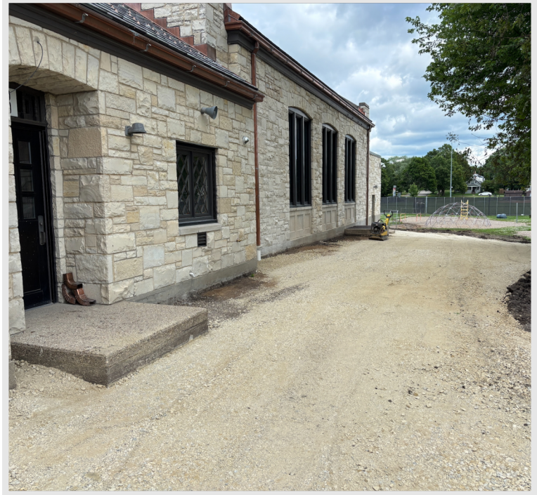
Site storm system replacement is complete on the south side of the building, and the base is graded/compacted for new sidewalks!
