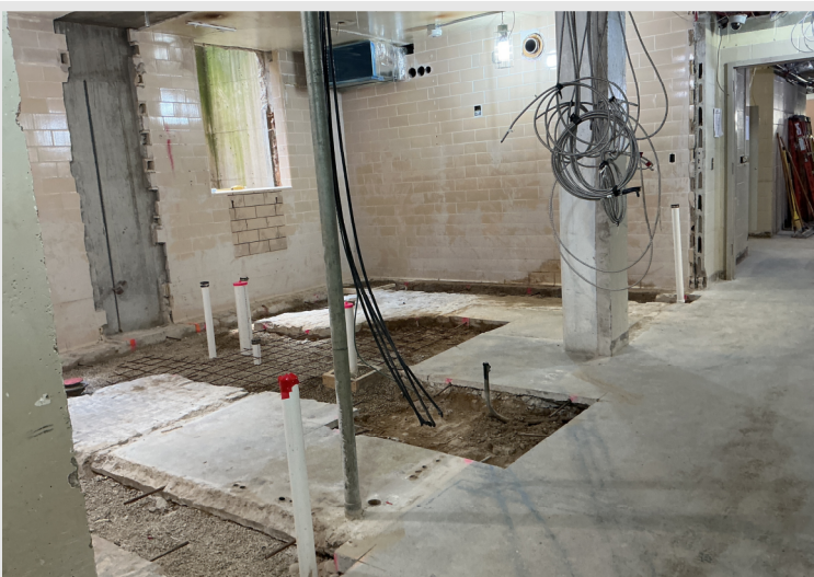
With the recent completion of the underground plumbing rough-ins and reinforcement in progress, the Lower-Level is almost set for new concrete!
