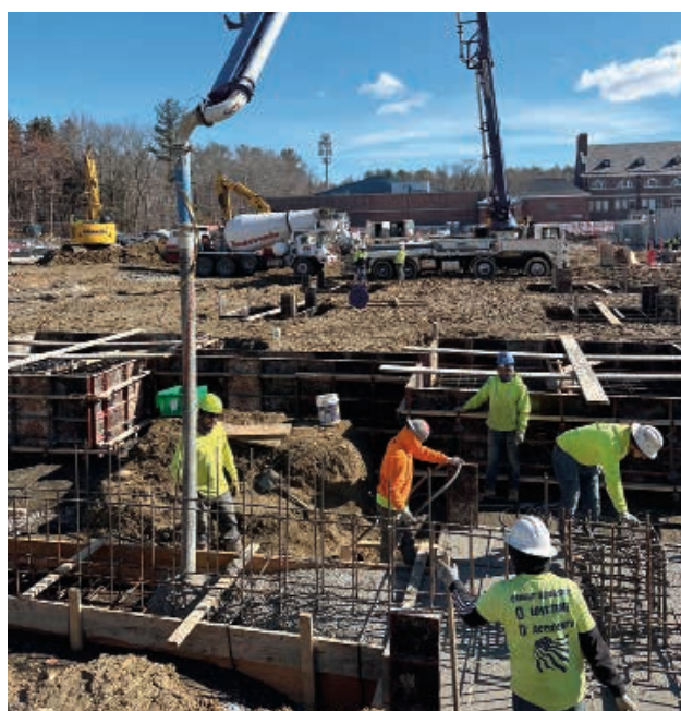
At the end of February, rebar was installed, so that concrete could be poured (below) onto the foundation and column support footings.
